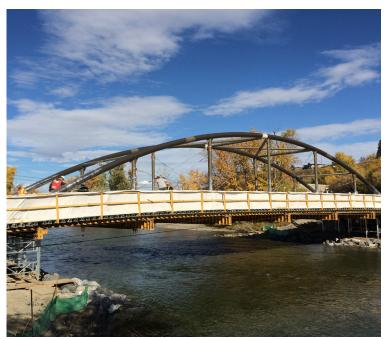
Together, the team determined that the preferred option should allow the arch to deflect under the weight of the wet concrete and for the concrete to cure its in-service profile.
