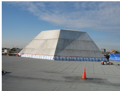
Aga Khan Museum roof construction: In order to support and build the double roofs while maintaining isolation, concrete was poured in sections, with neoprene isolators set between frames and formwork.
