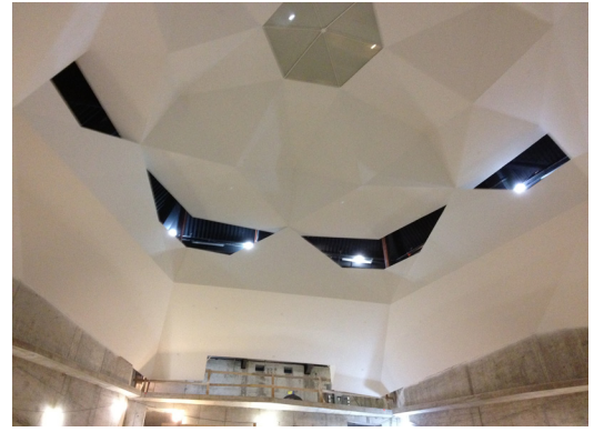
Above left: Aga Khan Museum Auditorium in construction. Above right: The Auditorium ceiling, kept as a symmetrical hexagon to serve the architectural vision and acoustic function.
