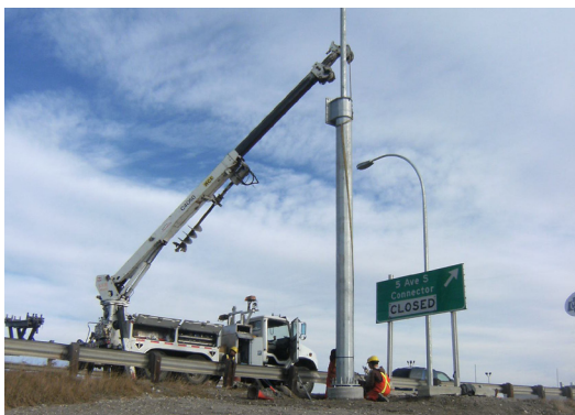
ACE Construction Erecting a Camera Tower
