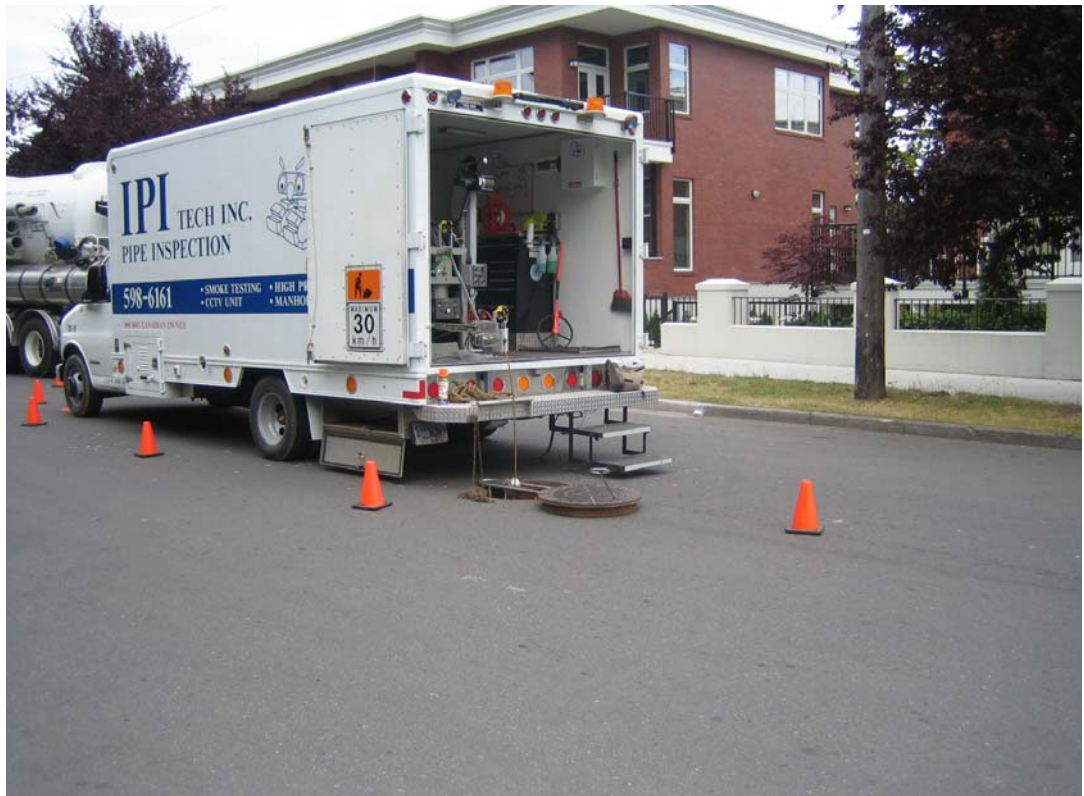
Photo 2: Using an innovative camera launched from this truck eliminated the need to inspect lateral sewers by either entering building or excavating.
