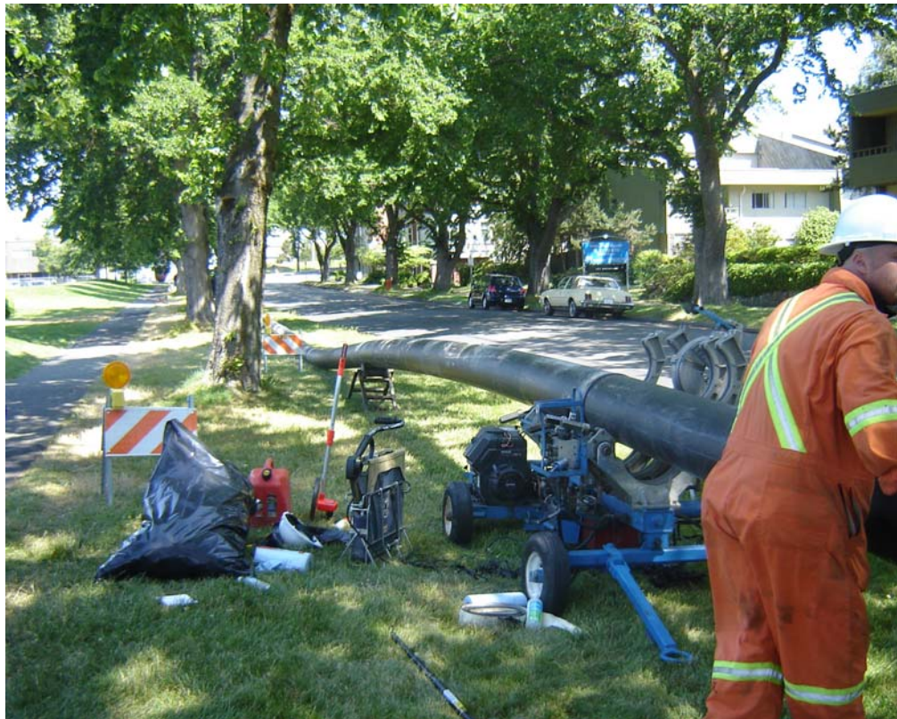
Photo 3: Fusing replacement pipe before trenchless installation
