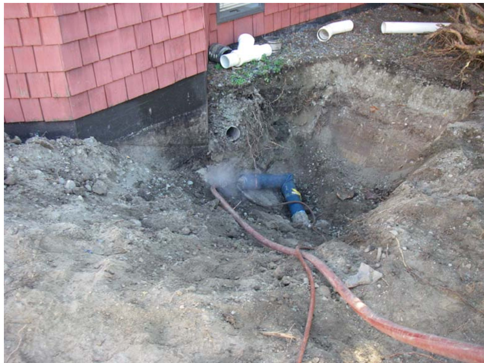
Photo 6: Rehabilitating a service lateral with CIPP (cured-in-place pipe)
