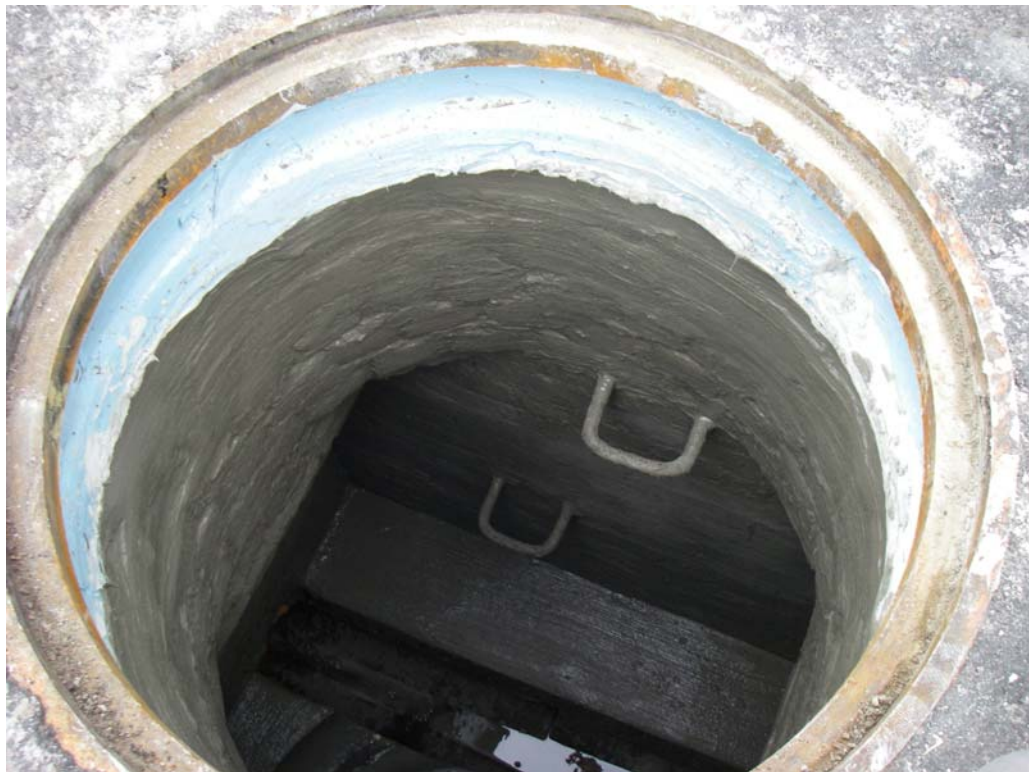
Photo 8: Manhole, with coating applied, after rehabilitation
