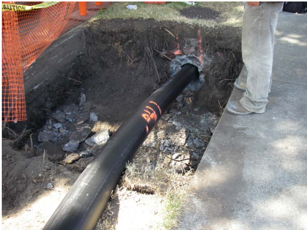
Photo 4: Pipe bursting entry pit
