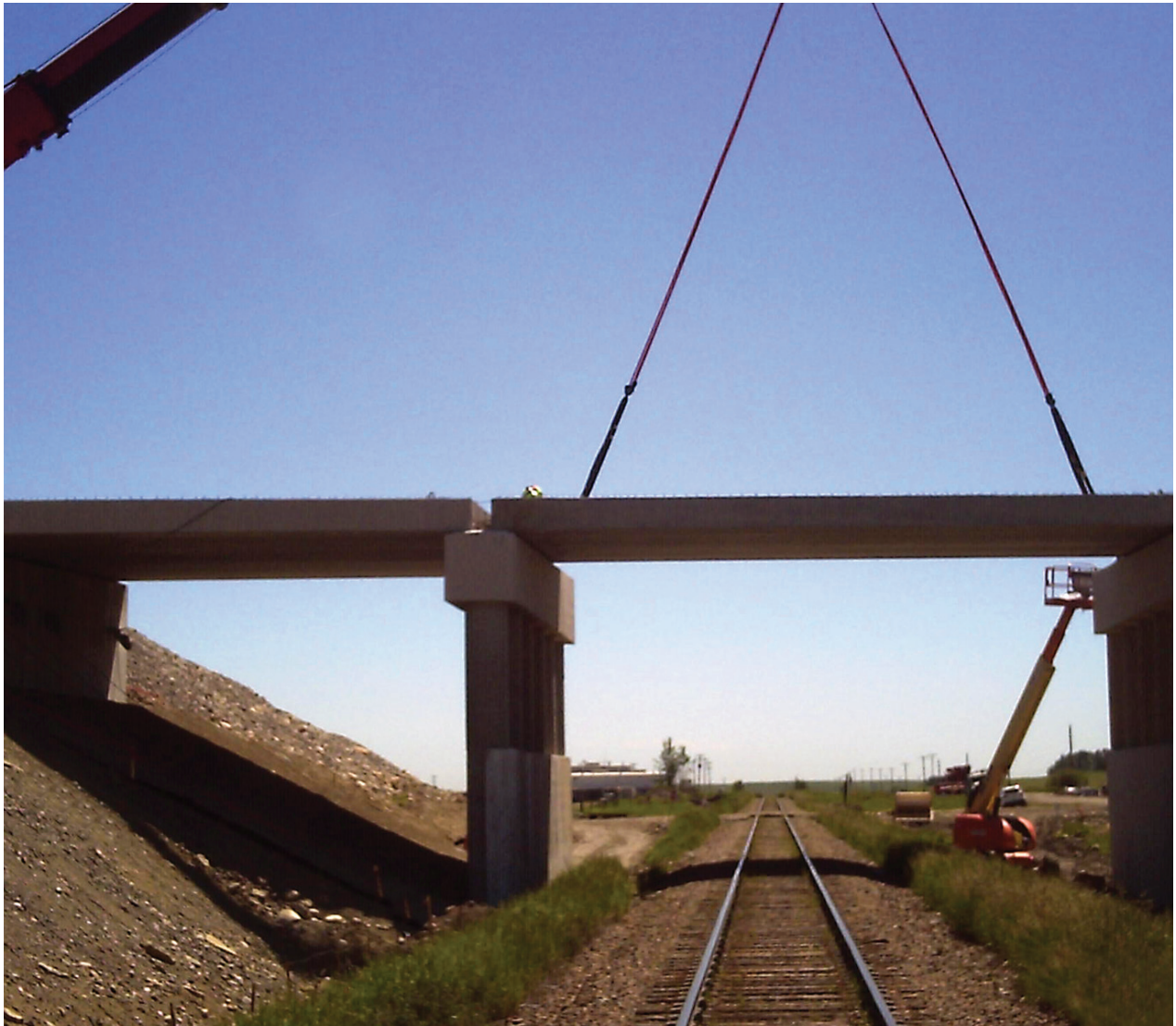
CPR Overpass Girder Erection
