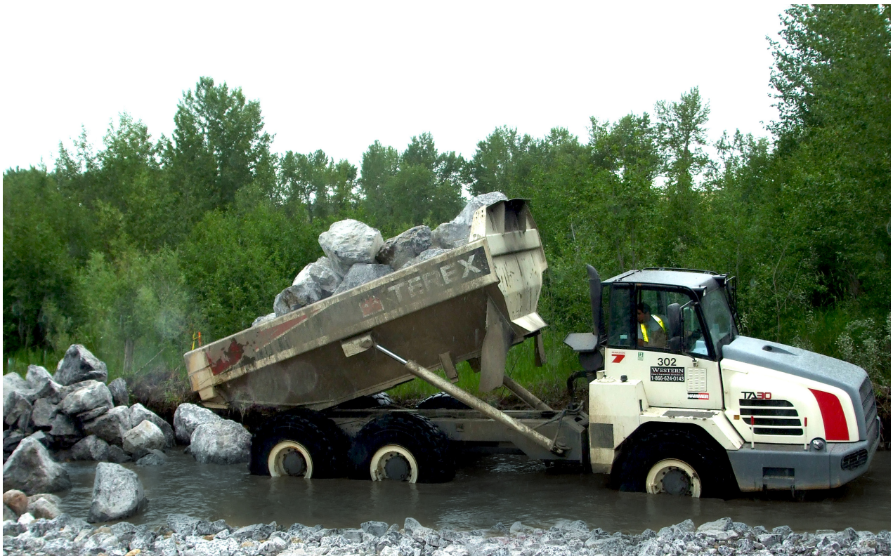
Constructing the River Guide Bank
