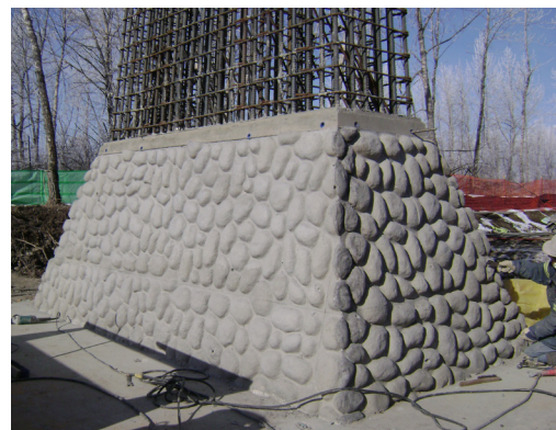
Pier Foundation Cast and Finished to Imitate Local Rock Boulders
