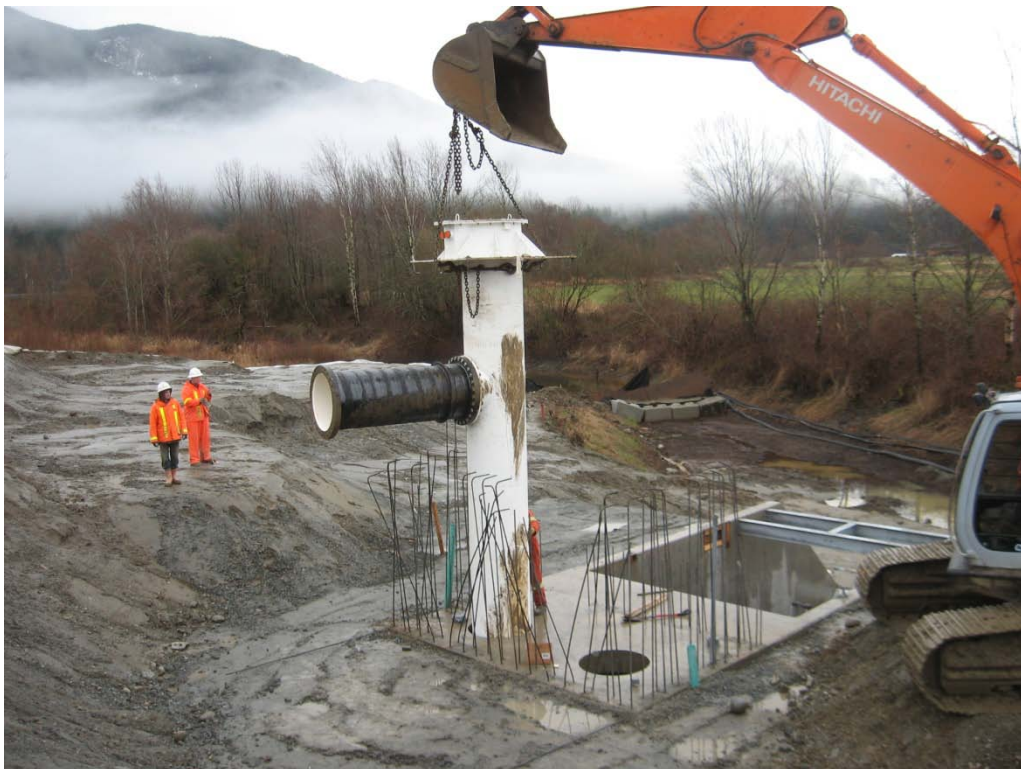
Installation of the drainage pump discharge columns. Drainage pumping capacity increased to 1,500 L/s.
