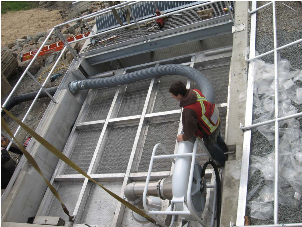
Submersible-centrifugal, hydraulic driven, fish-friendly transfer pump and discharge piping mounted integral to the fish screen.
