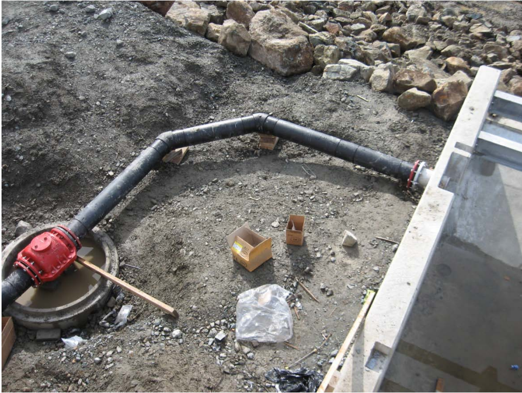
Fish discharge piping passes through a fish-friendly duckbill type check valve.
