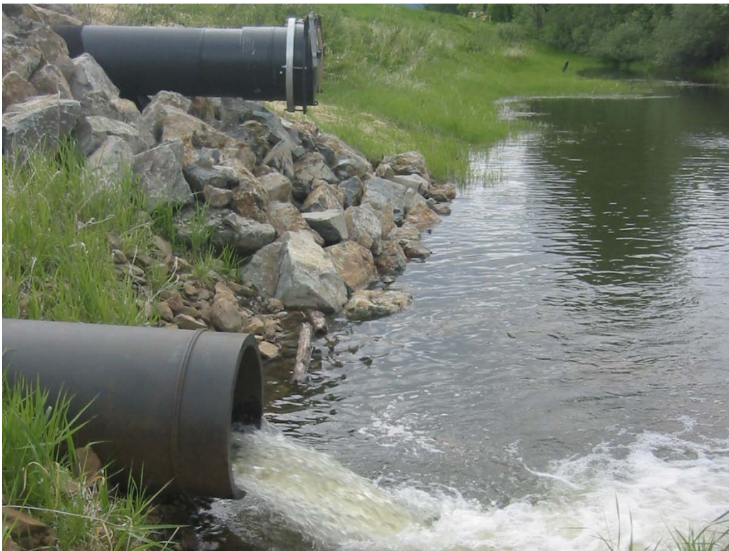
Dedicated pumped fish pipeline (foreground), and pumped drainage discharge pipes (background), discharging into a basin adjacent to the Harrison River.
