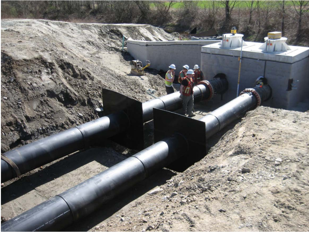
Installation of new 750 mm diameter HDPE drainage discharge pipes passing through the dike.
