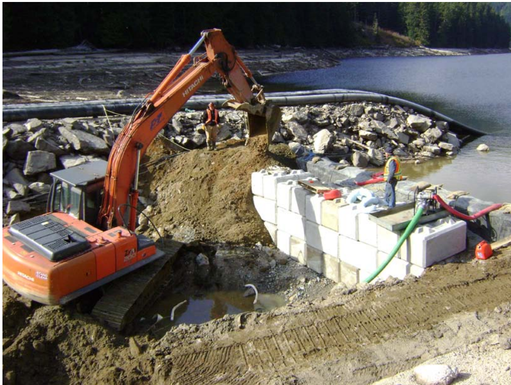
Photo 2: Construction of temporary lock-block dam to allow for work within the channel. Temporary bypass piping shown on far shore.
