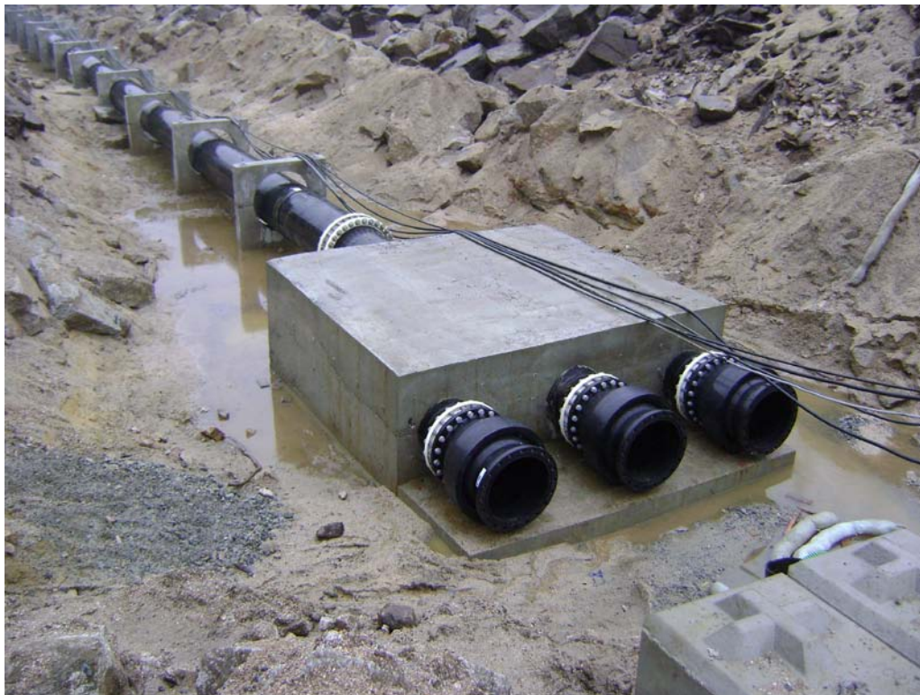
Photo 6: Pipe Header Block installed at the end of the channel with flexible ball joints allowing initial rotation of the 3 - 600 mm \varnothing pipes out to the floating pump station.
