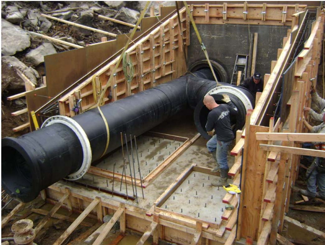
Photo 7: 900 mm ø Piping at Discharge Box: Check valve to be installed on Wye branch allowing gravity inflow during high water levels and pumped flow during low water levels.
