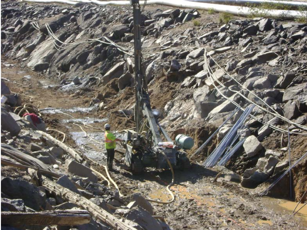
Photo 3: Drilling Rock Anchors in Channel: All equipment within channel used vegetable based drilling and hydraulic fluids to avoid contamination of waterway.
