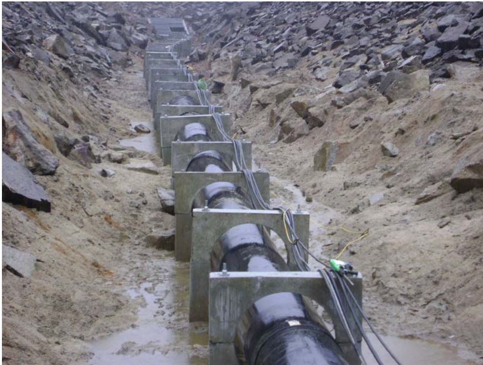
Photo 5: 900 mm \varnothing HDPE pipe installed in channel with concrete saddle supports and rock anchors to prevent pipe flotation while allowing thermal expansion/contraction of the HDPE pipe.
