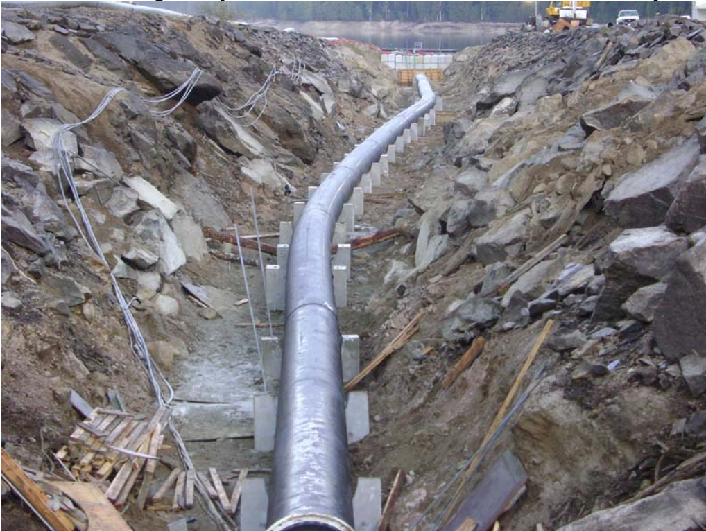
Photo 4: Installation of 900 mm ø HDPE pipe in dewatered channel after construction of temporary dam and rock anchor drilling.
