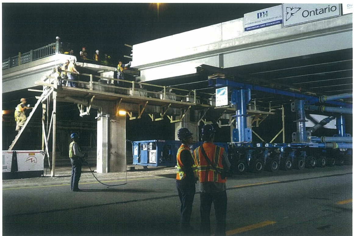
New Span 2 being moved into position using a SPMT
