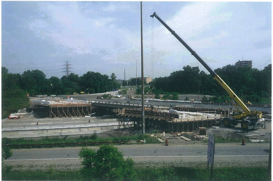
New Spans 1 and 4 casted by the side of the existing deck
