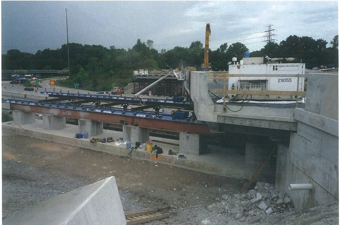
New Span 4 being moved into position using Jack and Slide method PHOTO CREDIT: Morrison Hershfield
