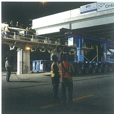
New Span 2 being installed with SPMT
