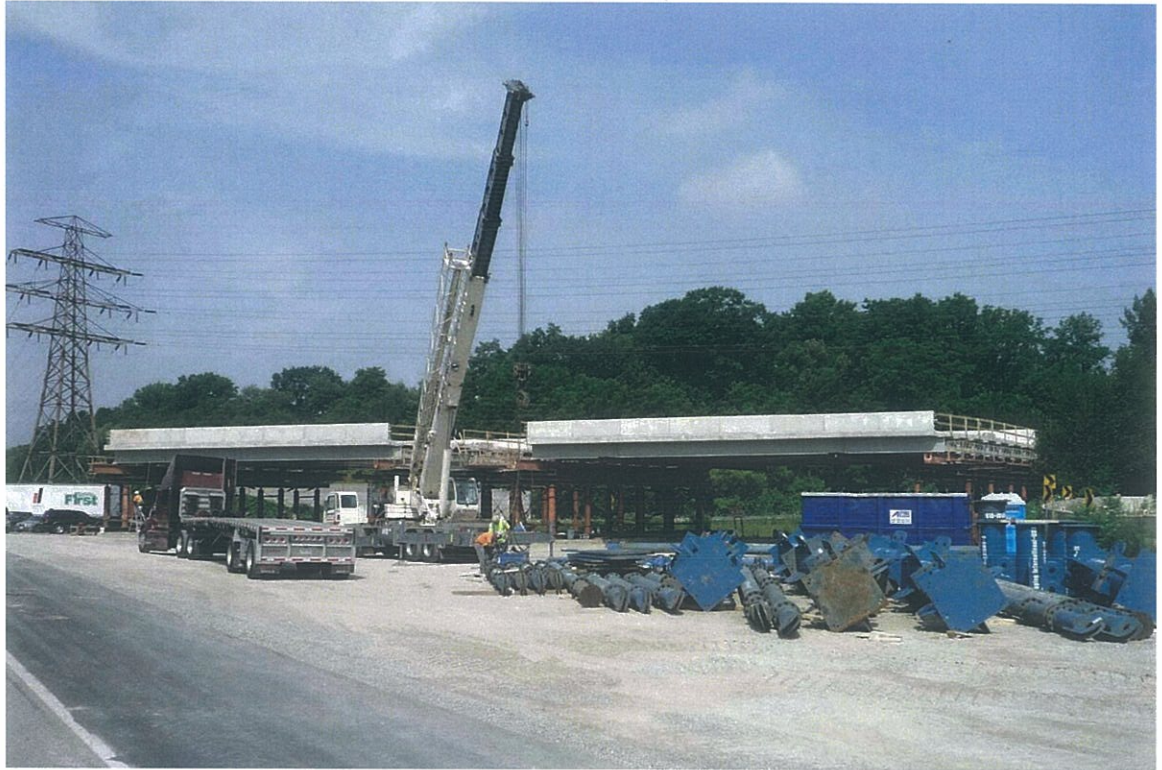
New Spans 2 and 3 prefabricated in Staging Area
