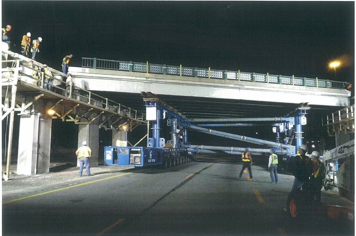
Existing Span 2 being moved away using a Self Propelled Modular Transporter (SPMT)
