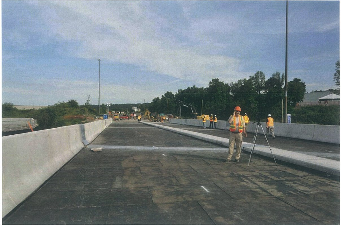
Final installation of waterproofing and paving
