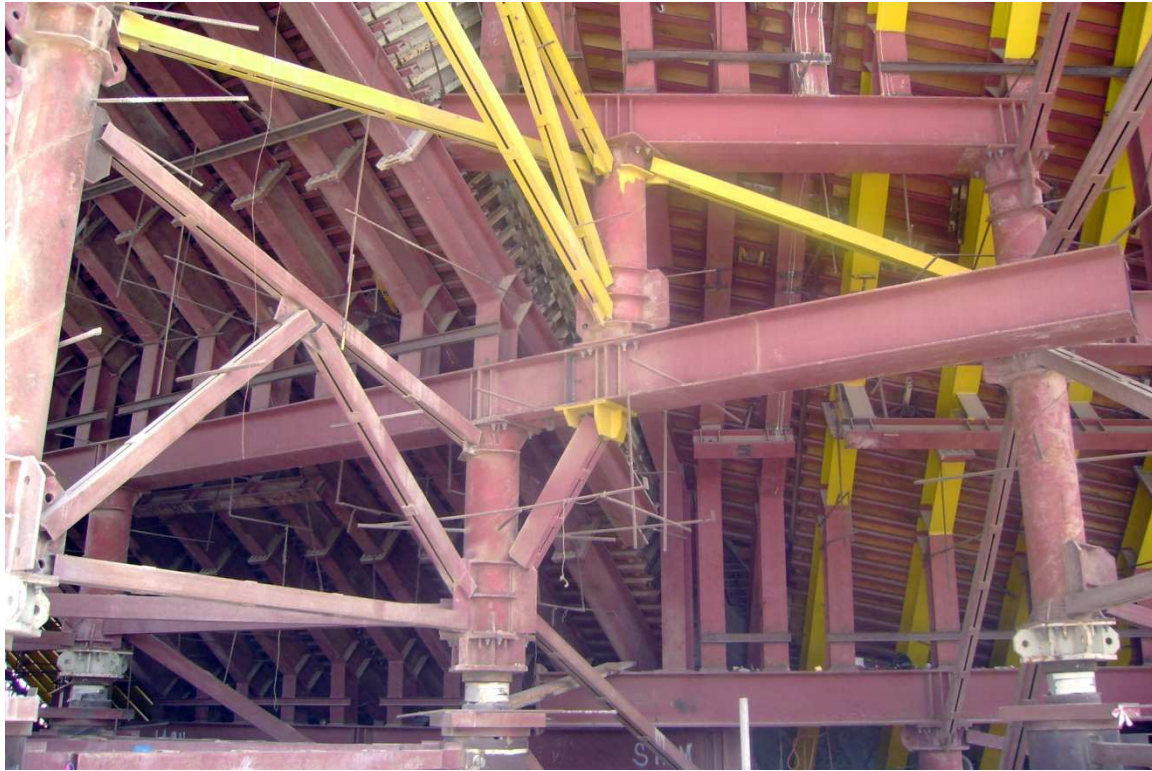
A typical detail of temporary formwork supports
