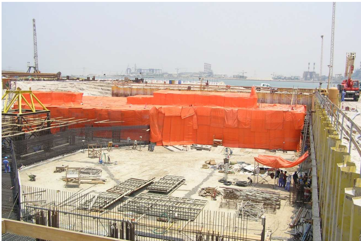
Insulation to keep the mass concrete warm in temperatures up to 50 °C
