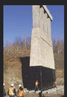
The structural system adopted by CIMA+ provided good energy dissipation through the placement of plastic hinges in the pier's ductile upper section, while keeping displacement at the top within acceptable limits.
