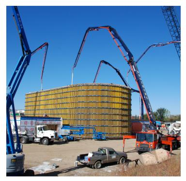
The wall was cast on October 1, 2009. The weather forecast was monitored closely to ensure that rain or cold temperatures would not adversely affect the pour. A backup pour date had been arranged in case of threatening weather. Concrete was placed simultaneously by four concrete pump trucks, ensuring a uniform rate of concrete placement around the perimeter of the chapel. A fifth pump was set up on standby in case of failure of one of the primary pumps, but was not required.
