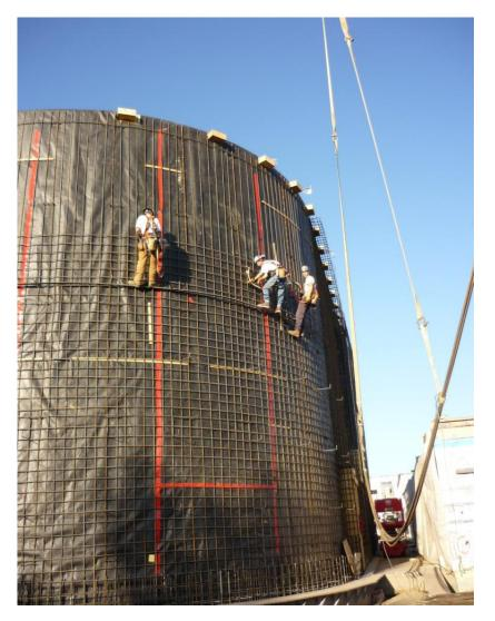
Reinforcing was chaired and tied only to the outside face of the wall so that no wire or chairs would be visible on the interior concrete surface. The inside face of the formwork was erected first, allowing rebar to be tied in place before "buttoning up" the outside form. During rebar placement, the formply on the inside face of the wall was protected from accidental damage by full height woven geotextile fabric.
