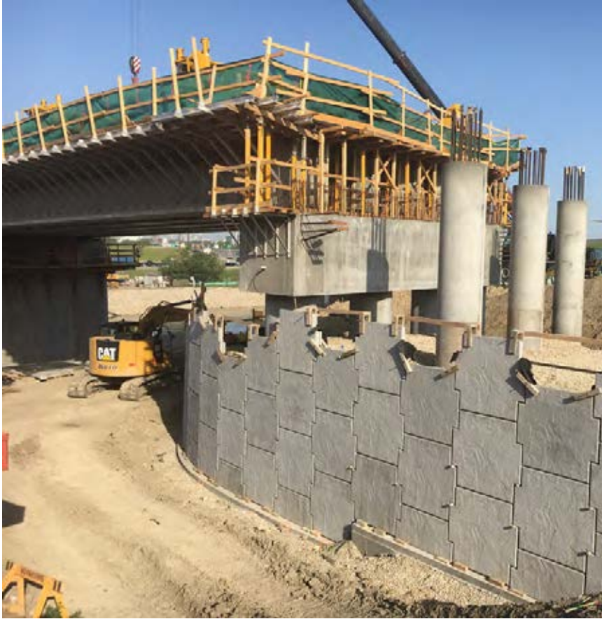
← Building retaining wall for the Western Headworks Canal bridge
