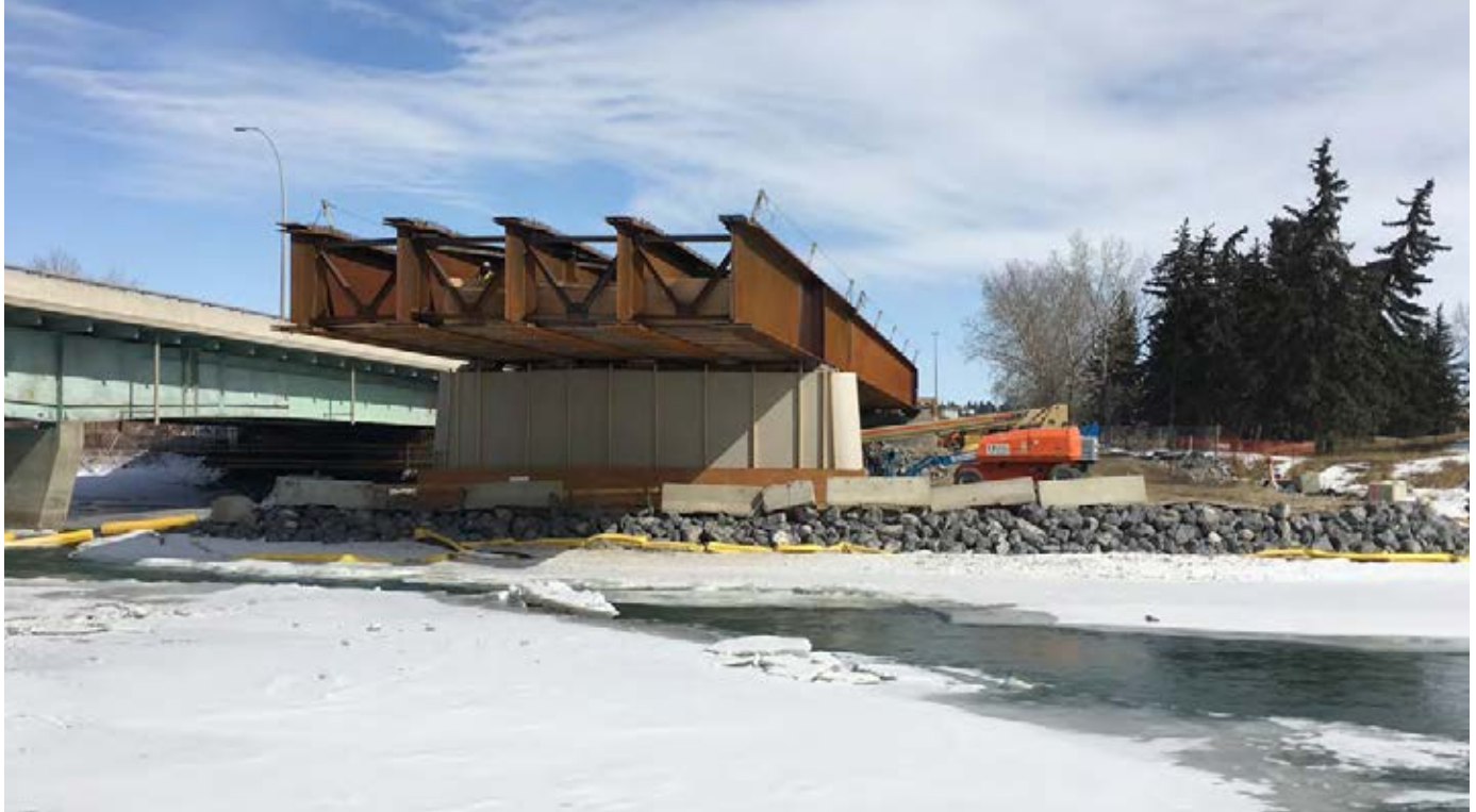
Bow River Bridge girders partially erected
