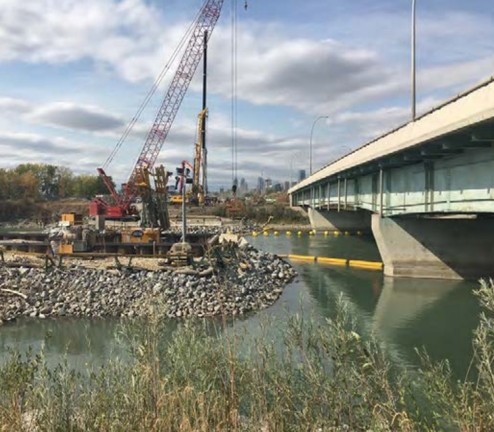
Bow River Bridge foundation construction work
