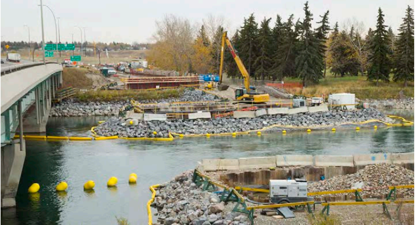
Bow River Bridge in-river foundation work
