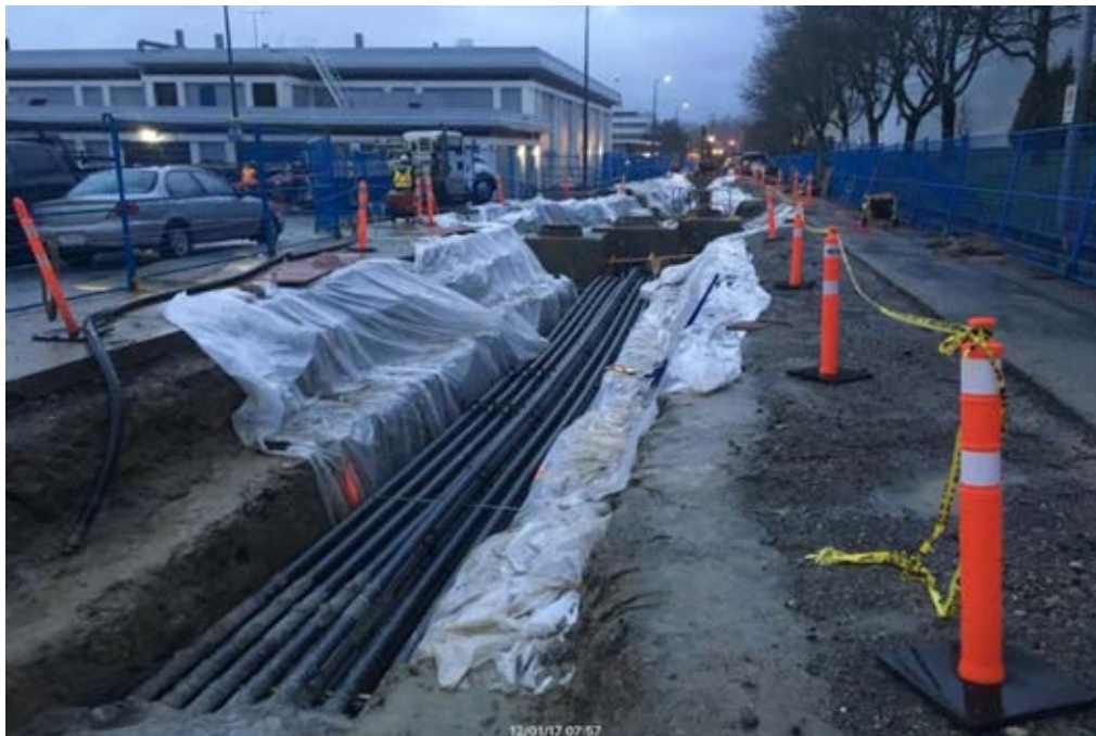
Photo 2: Carey Avenue electrical duct bank and manholes
