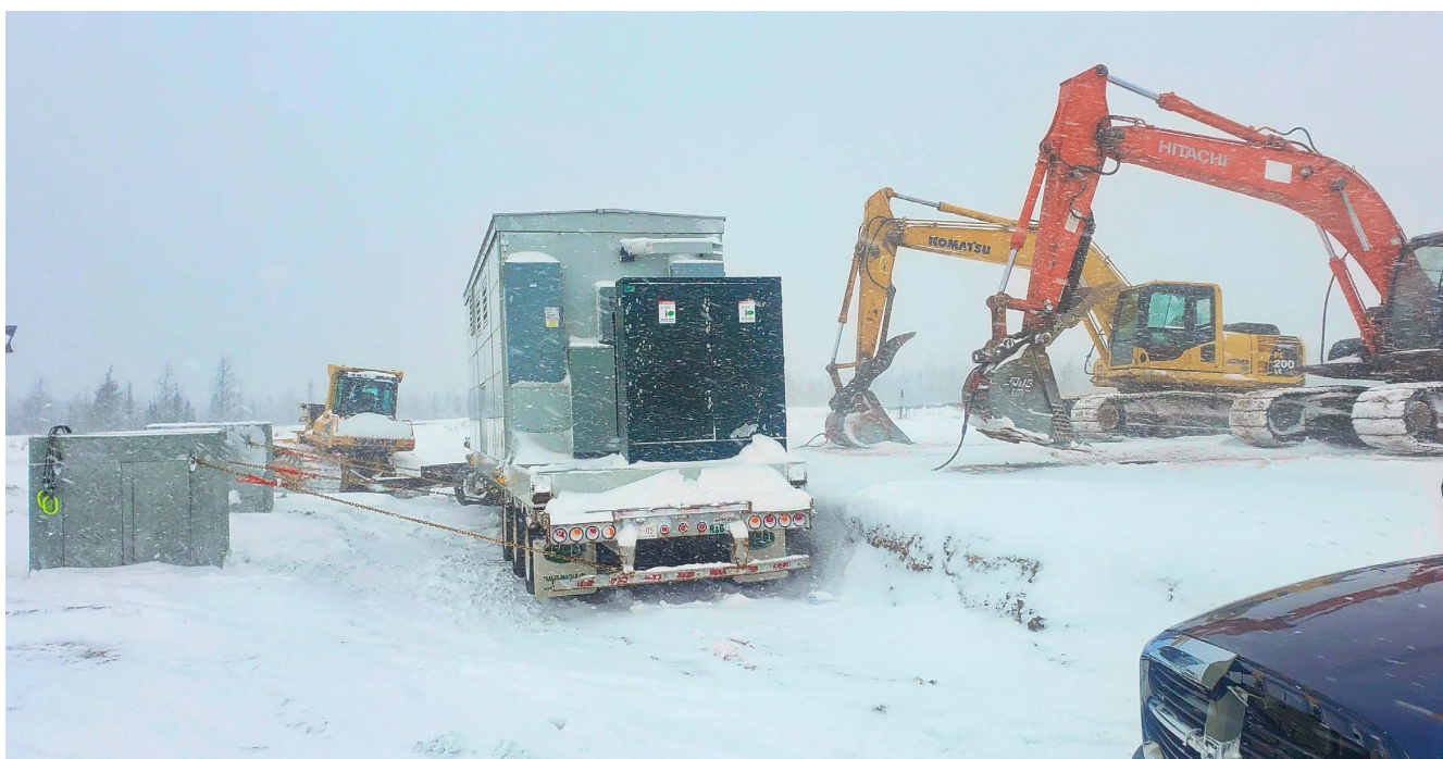
FIGURE 3: E-house dragging technique.
