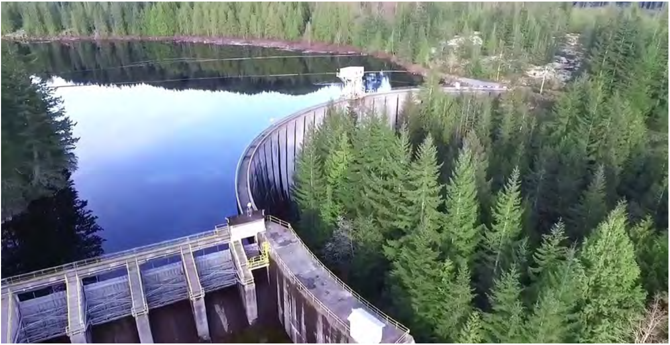
Overview of the Lois Lake Dam facilities
