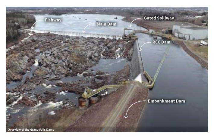
A key to the success of the new concept was the application of advanced hydrotechnical principles that demonstrated that the ten inflatable gates that had been thought to be required could be replaced with a simple overflow weir constructed immediately downstream of the existing spillway. This enhanced stability, provided the required discharge capacity and eliminated in-water work, thereby reducing environmental impacts. As part of the design,
