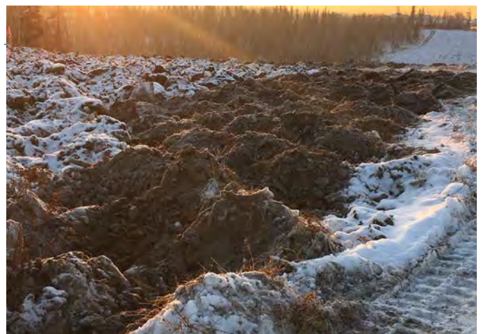
Surface roughening soil treatment at Conn Creek Ravine site
