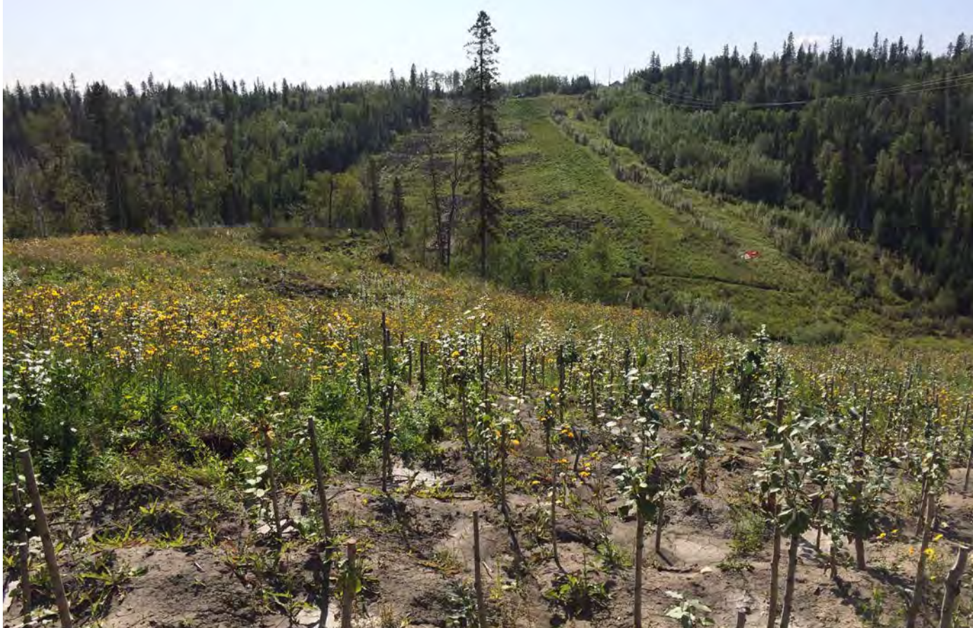
Conn Creek Ravine after bioengineering treatment
