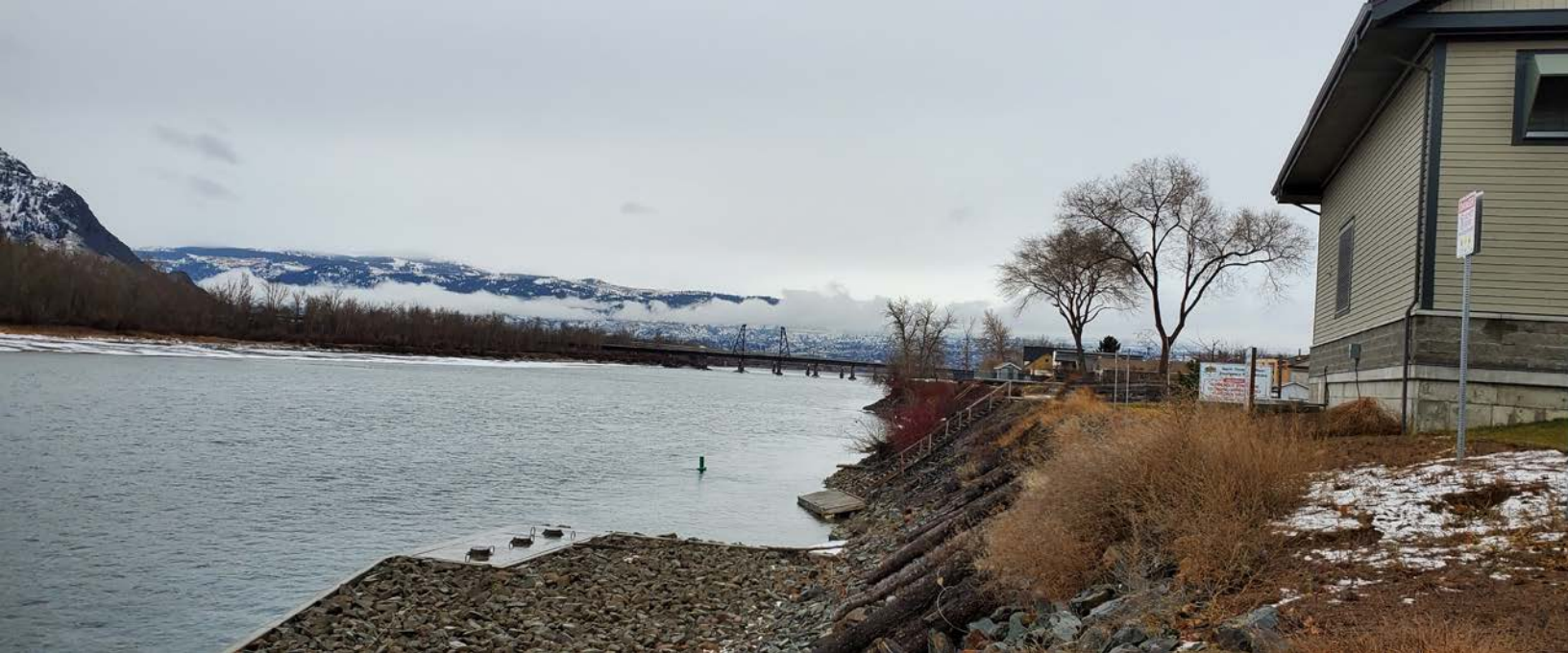
Gravity intake from the North Thompson River to the pumphouse
