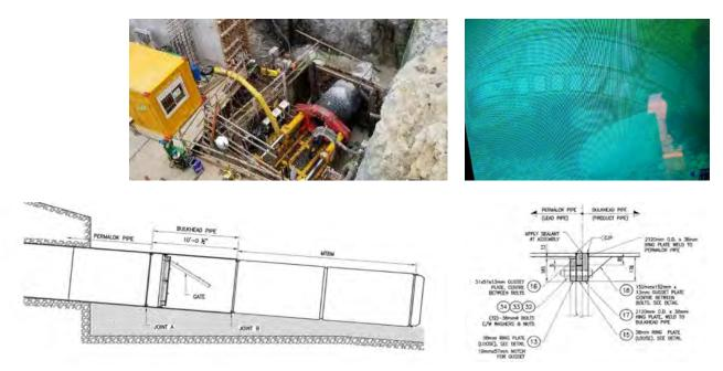
The inshore section from the new treatment plant to the ocean consisted of a 120-metre long, "wet-exit" microtunnelling drive which was constructed with a 2120-millimetre steel pipe section with a 25-millimetre pipe wall thickness to safely resist installation jacking forces. The pipe was driven through highly abrasive granodiorite bedrock.
