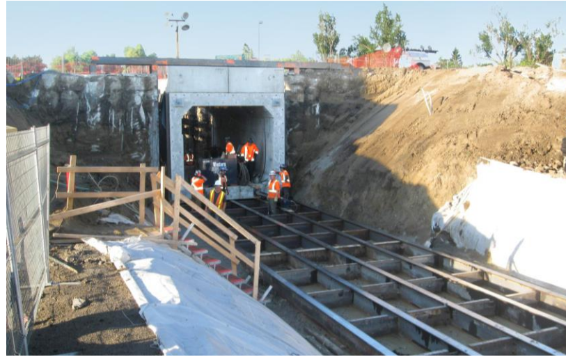
Jack and Slide tunnel installation
