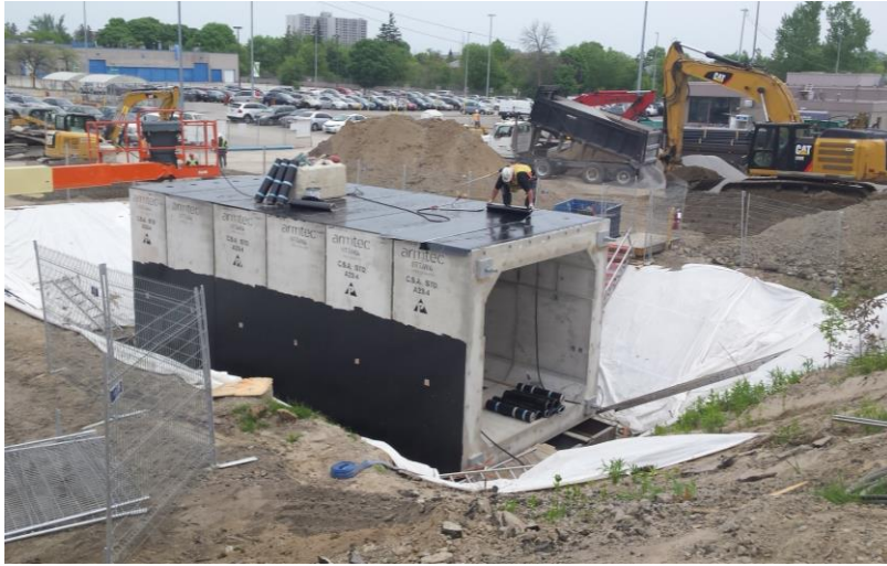
Precast tunnel segments installation
