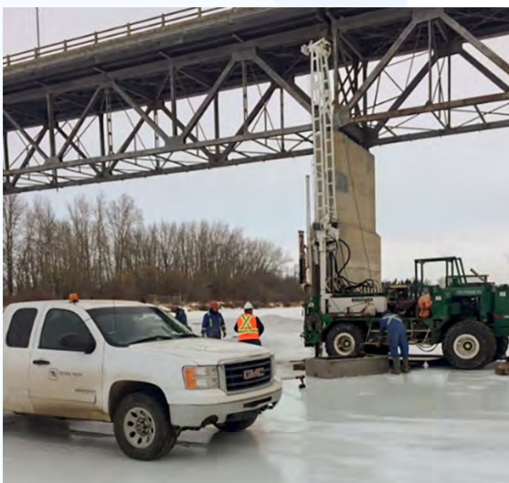
>> Ice Bridge for Geotechnical Investigations, February 2018
