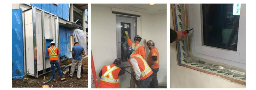
High performance triple glazing in Passive House certified window frames and curtain walls.
