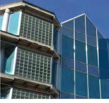
The existing Building NX was suffering from air infiltration, water penetration and condensation issues.
