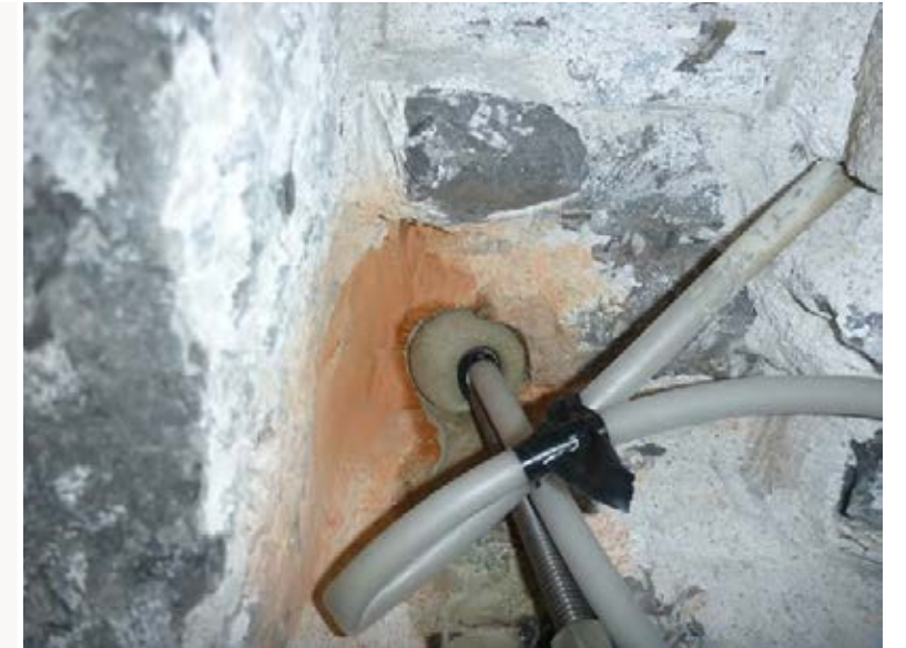
▲ Grouted anchors were used to reinforce masonry wall for seismic forces.
