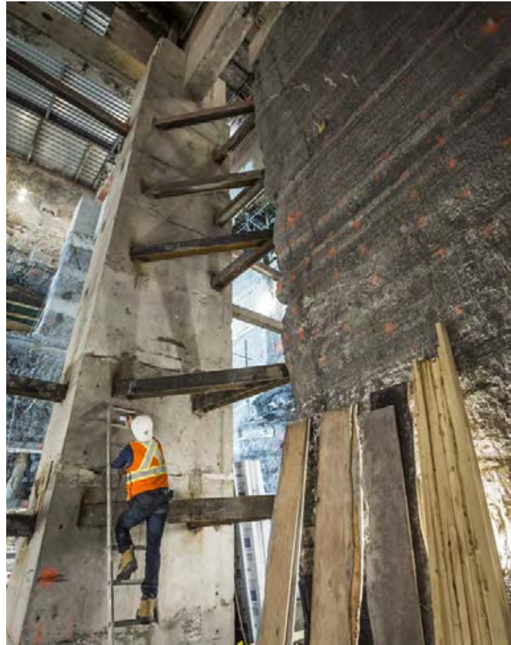
▲ Excavation Under Existing North Wing Building Above
