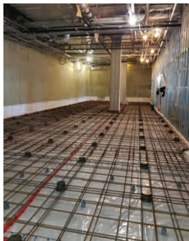
Floating floor being laid down
