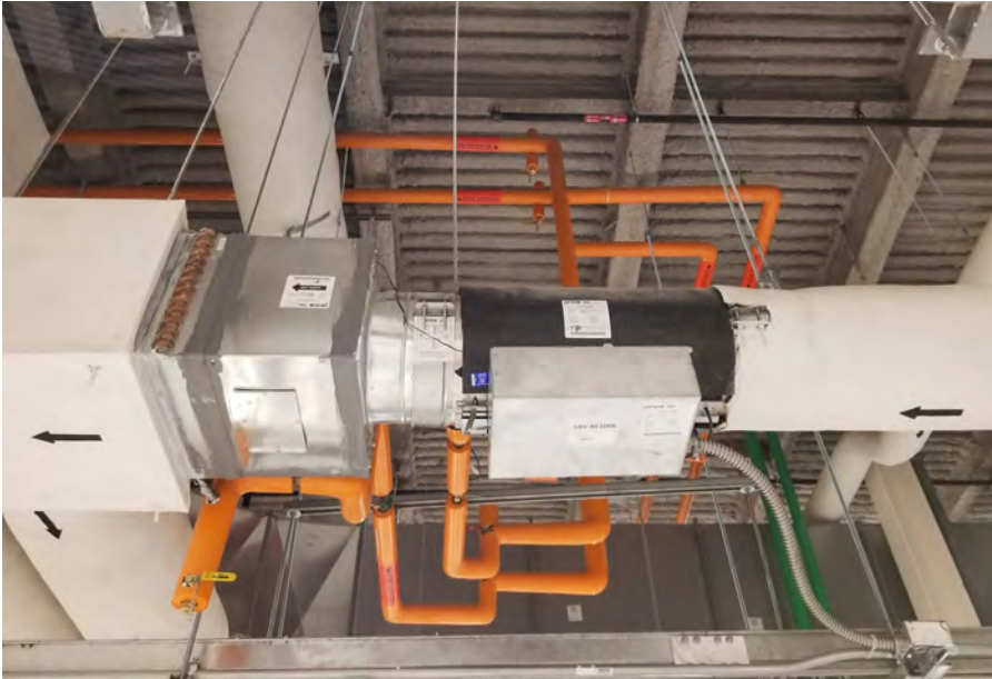
Venturi-Style Air Valve with Silencer and Reheat Coil
