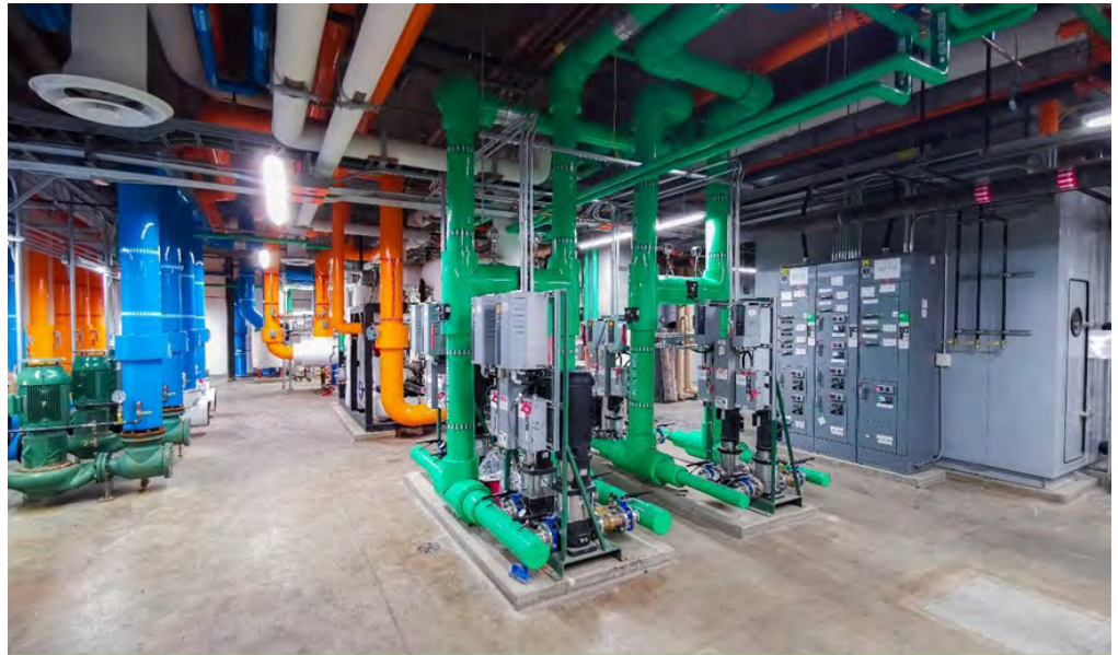
Steam, Hydronic & Domestic Systems Color-Coded for Ease of Identification
