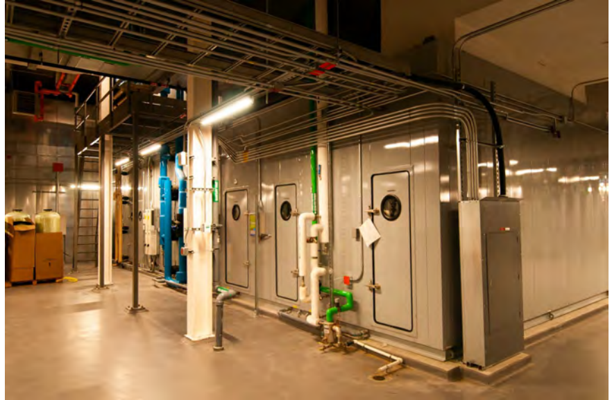
One of seven (7) central station air handling units
