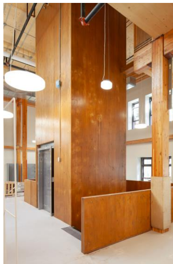
CLT Elevator Core. Photo Credit Scott Norsworthy
