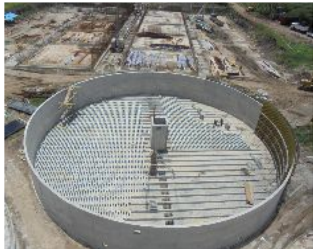
>> Trickling Filter - Filter block placement
