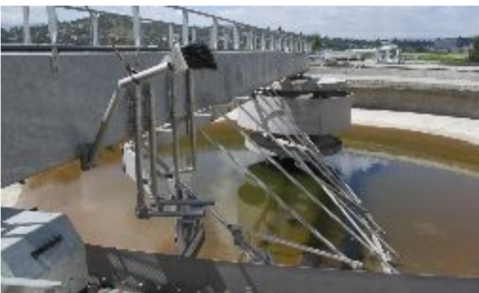
>> Secondary Clarifier - Rotating Arm
