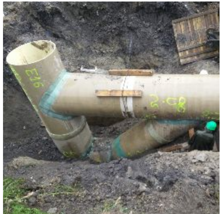
>> Man hole drop structure
