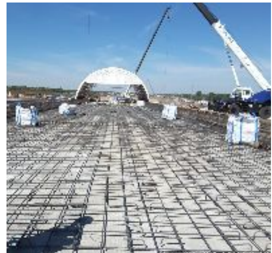
Bridge Reinforcement Inspection on Structure 1 over PTH59
