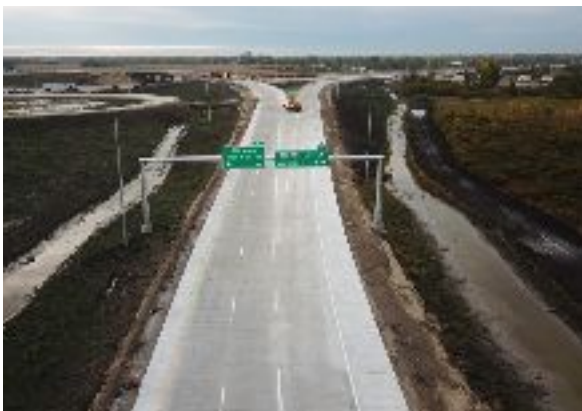
Westbound-Northbound/Southbound Ramp from PTH101 to PTH59
