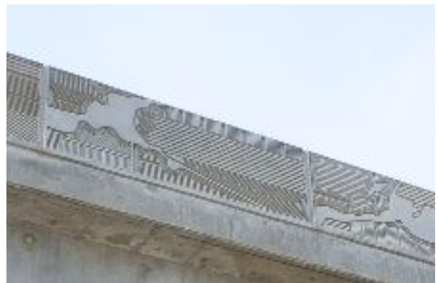
Aesthetic Treatment on Structural Barriers
