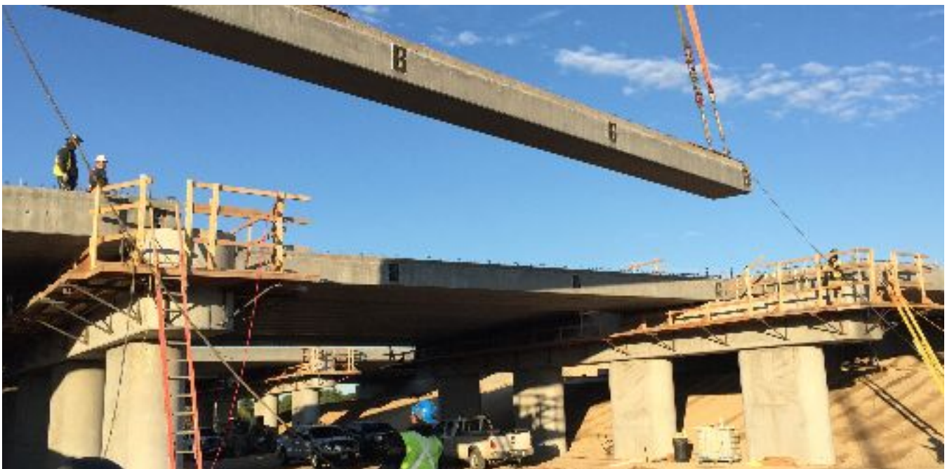
Girder Erection
