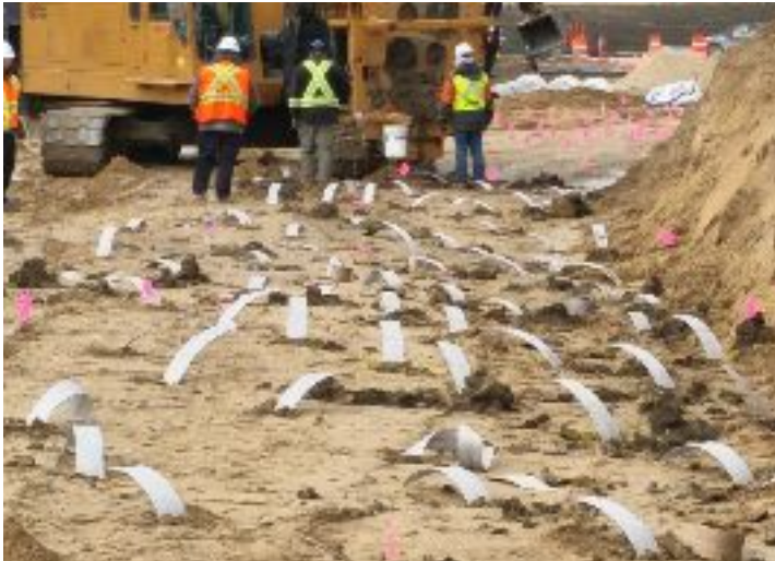
Wick Drain Installation
