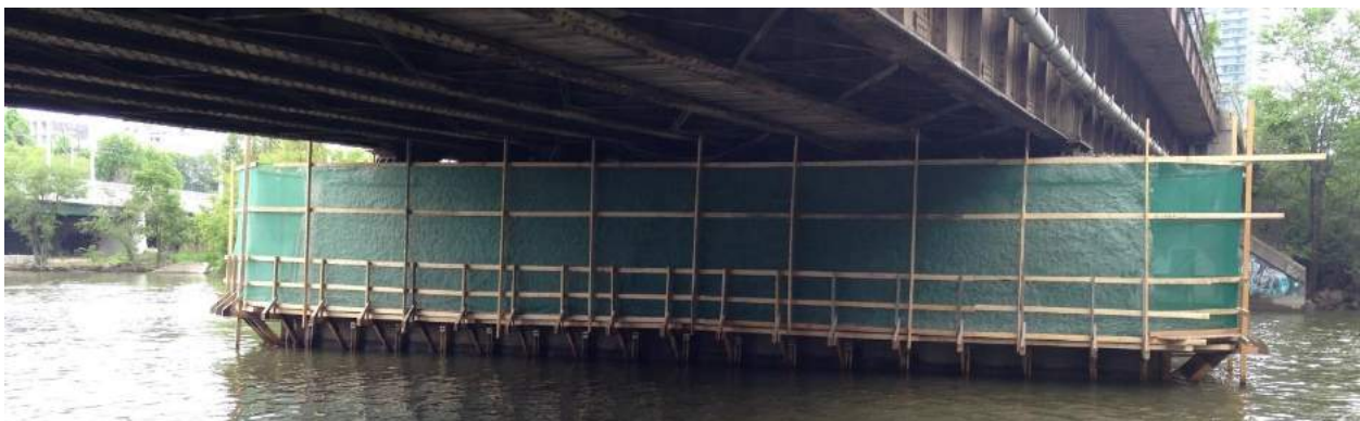
Figure 3: Environmental protection installed around the center pier for concrete chipping.
