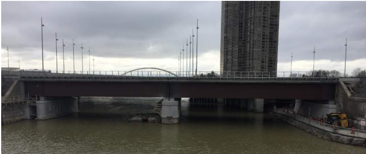
Figure 2: Humber River Bridge with all 8 spans replaced and open for service.
