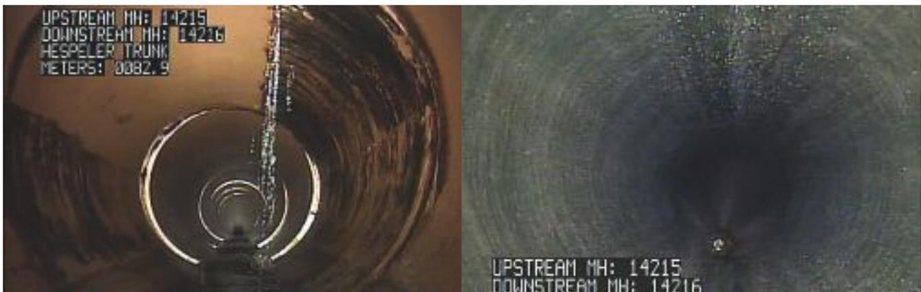
*Pre- and post-lining view of pipe with longitudinal cracking and running infiltration*
