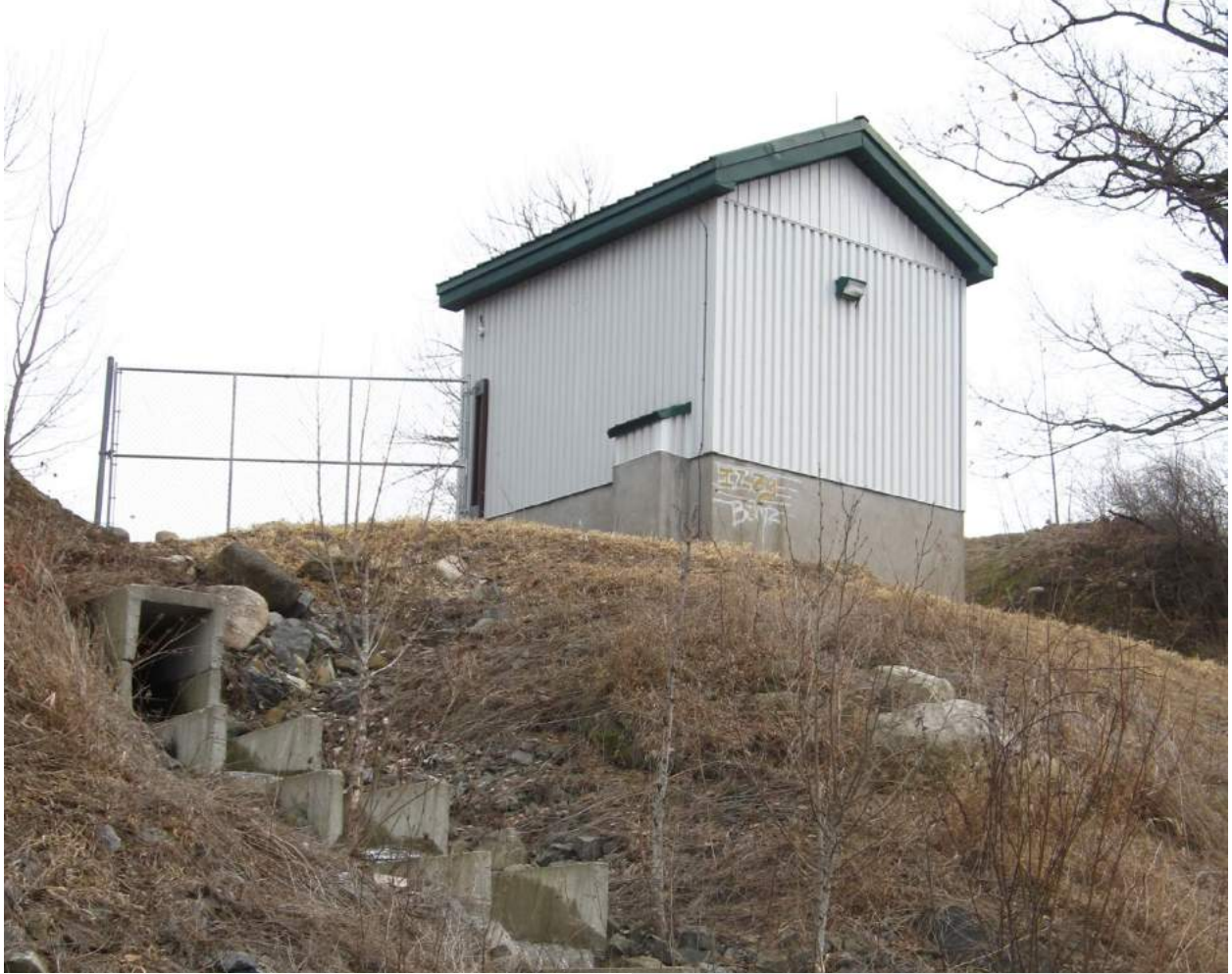
Mohawk Council of Akwesasne water intake.
