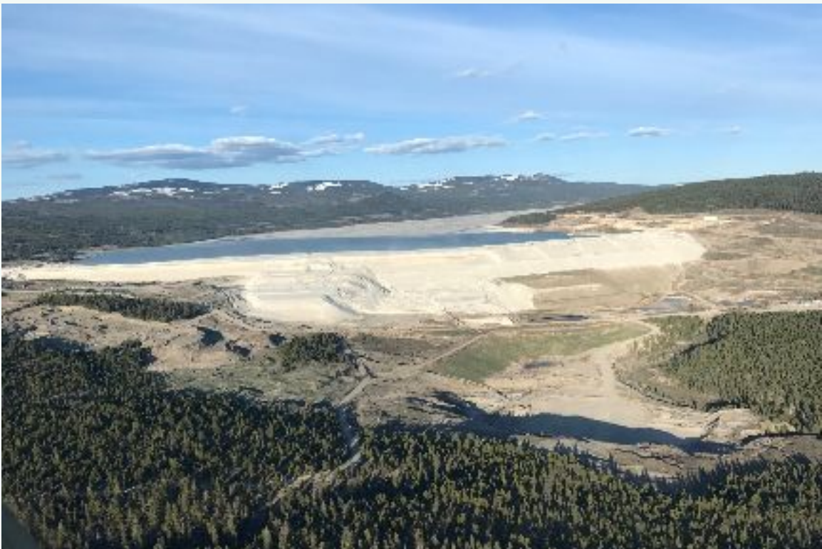
Highland Valley Copper, BC, Canada
