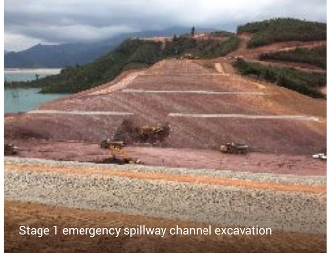
Stage 1 emergency spillway channel excavation
