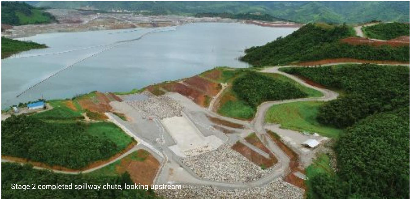
Stage 2 completed spillway chute, looking upstream
