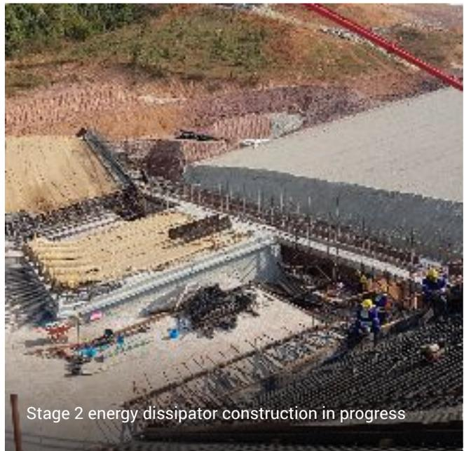
Stage 2 energy dissipator construction in progress
