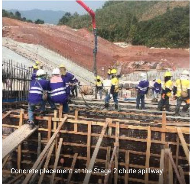
Concrete placement at the Stage 2 chute spillway
