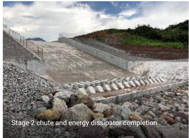
Stage 2 chute and energy dissipator completion
