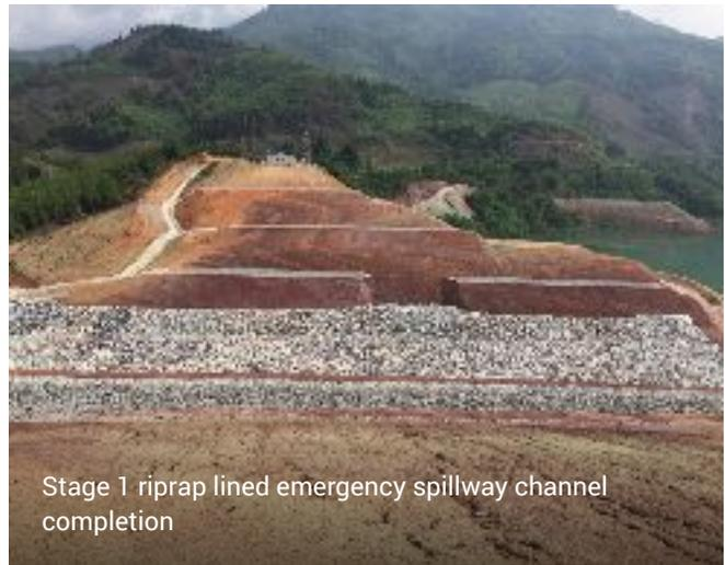
Stage 1 riprap lined emergency spillway channel completion
