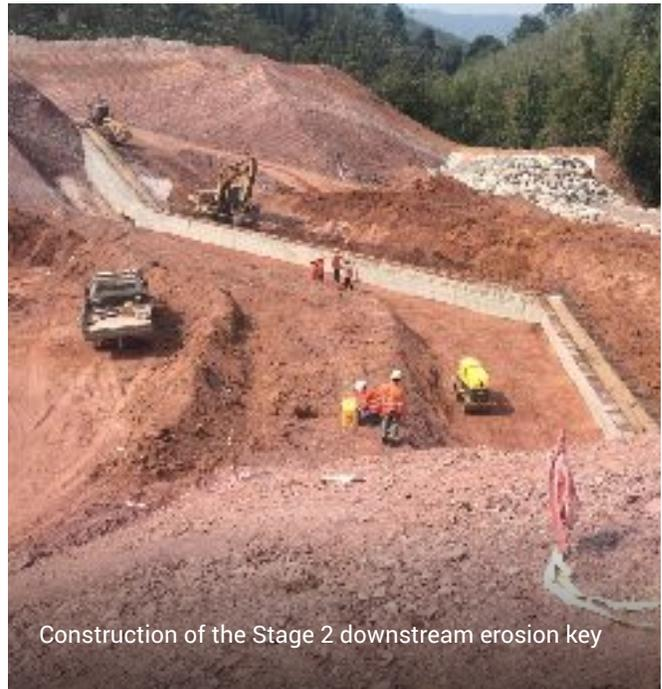
Construction of the Stage 2 downstream erosion key
