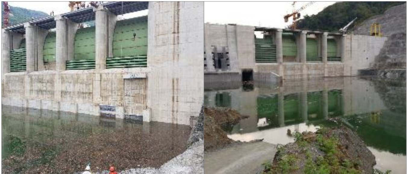
Diversion conduit closure (left) and dam before impoundment (right)
