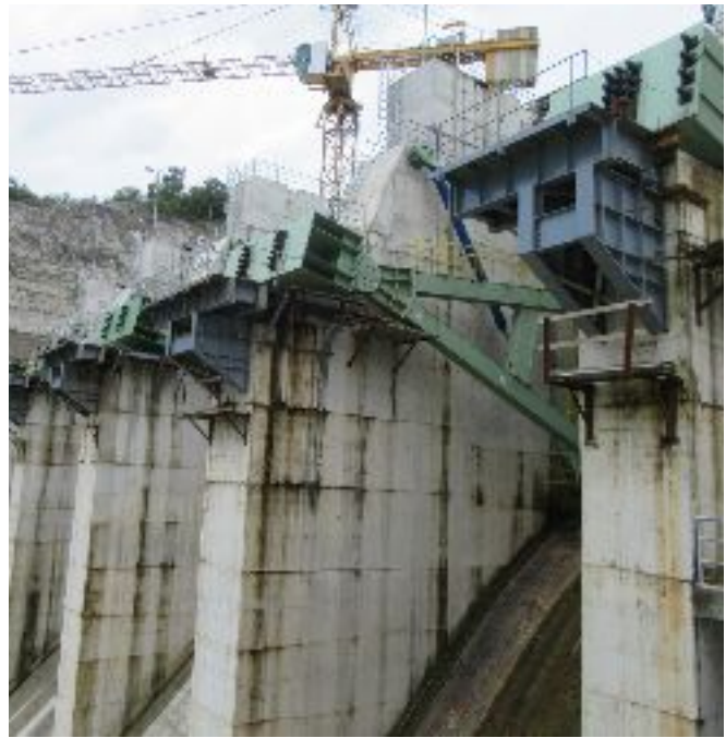
Gate trunnion support structure and anchorage
