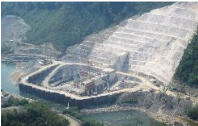
Stage 1 cellular cofferdam
