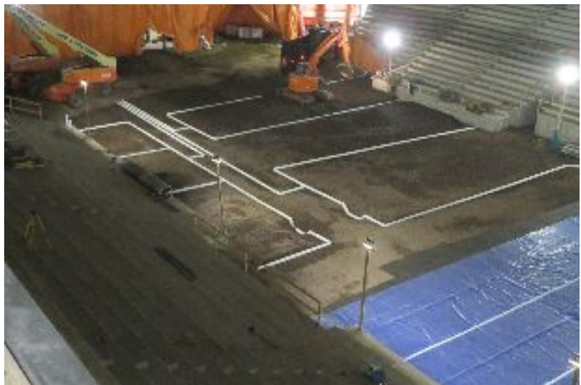
Installation of subfloor vapour intrusion mitigation system under the ice surface
