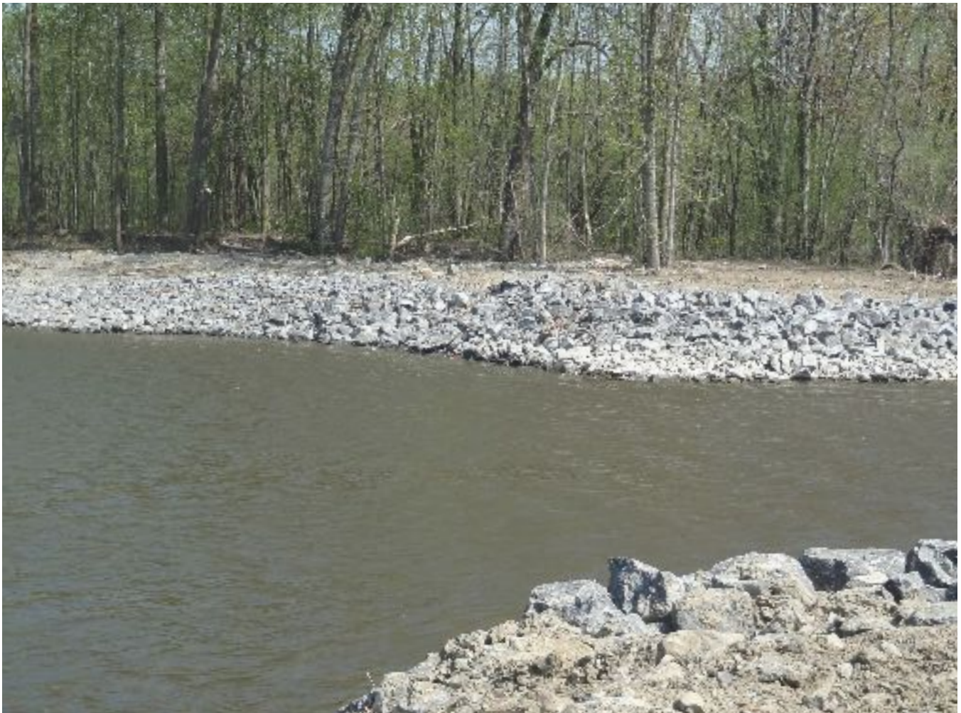
Shoreline after remediation
