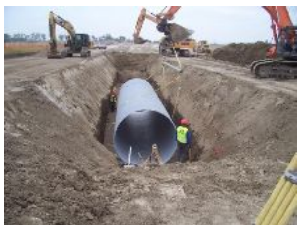
First Pipe Being Installed
