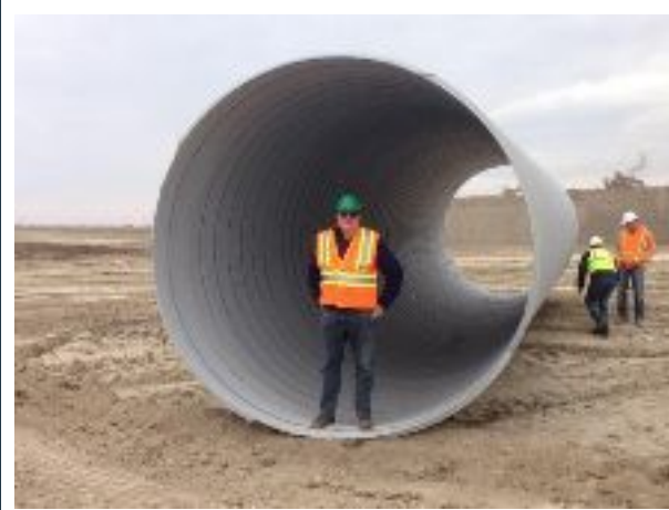
First Pipe Delivered to Site
