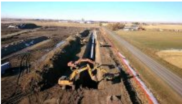
Aerial View of Syphon Installation Along 43 rd St.
