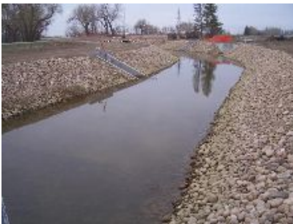
Approach Canal to Syphon Inlet Structure
