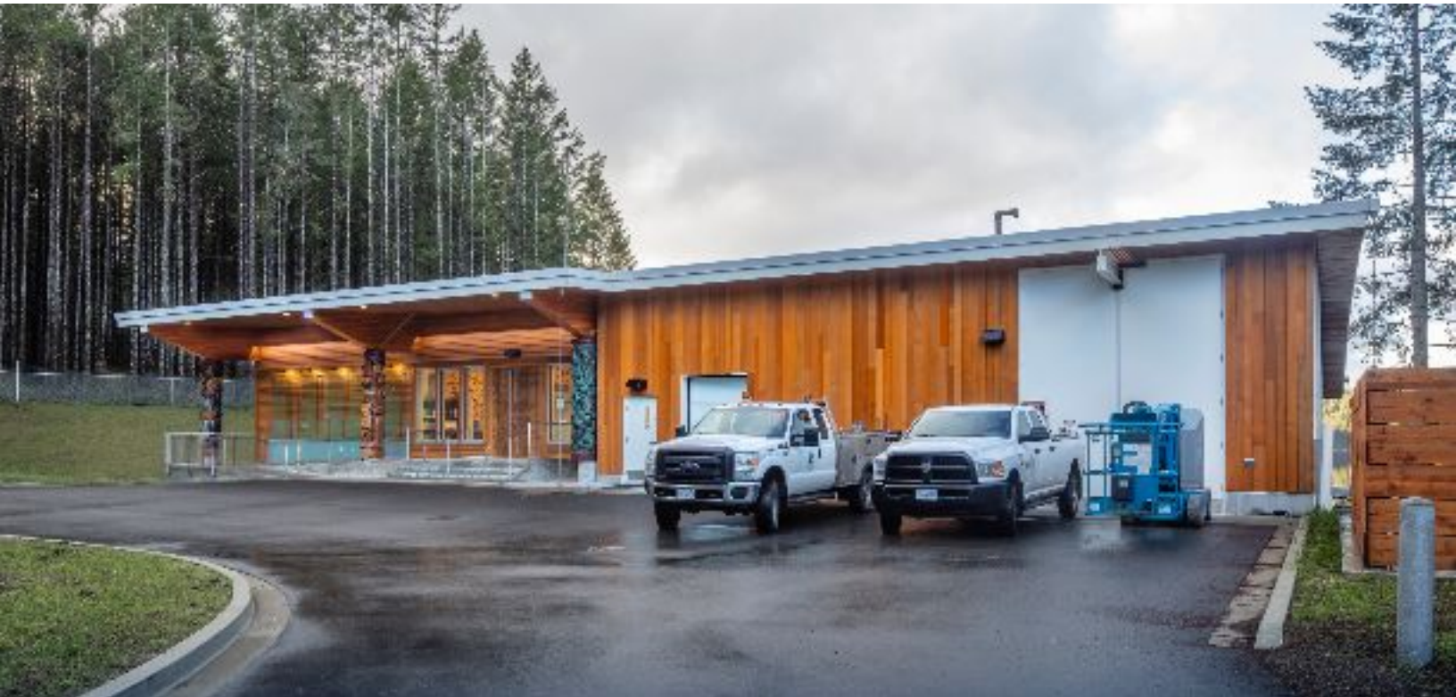
The exterior design of the Campbell River Water Supply Centre, which was a collaboration between Stantec, the City, and the Wei Wai Kum First Nation band
