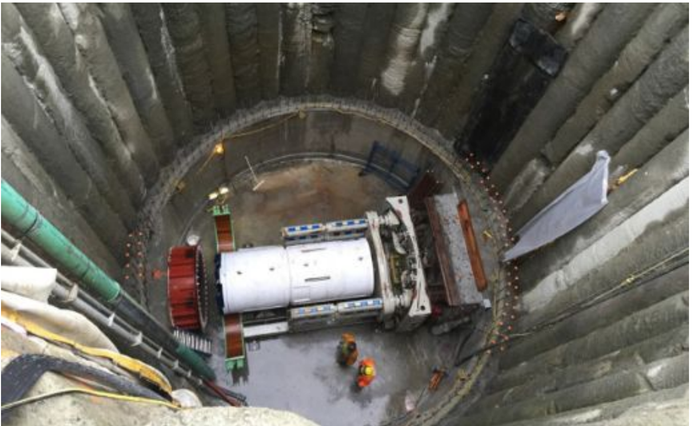
15.2m deep caisson to accommodate the vertical turbine pumps and shafts
