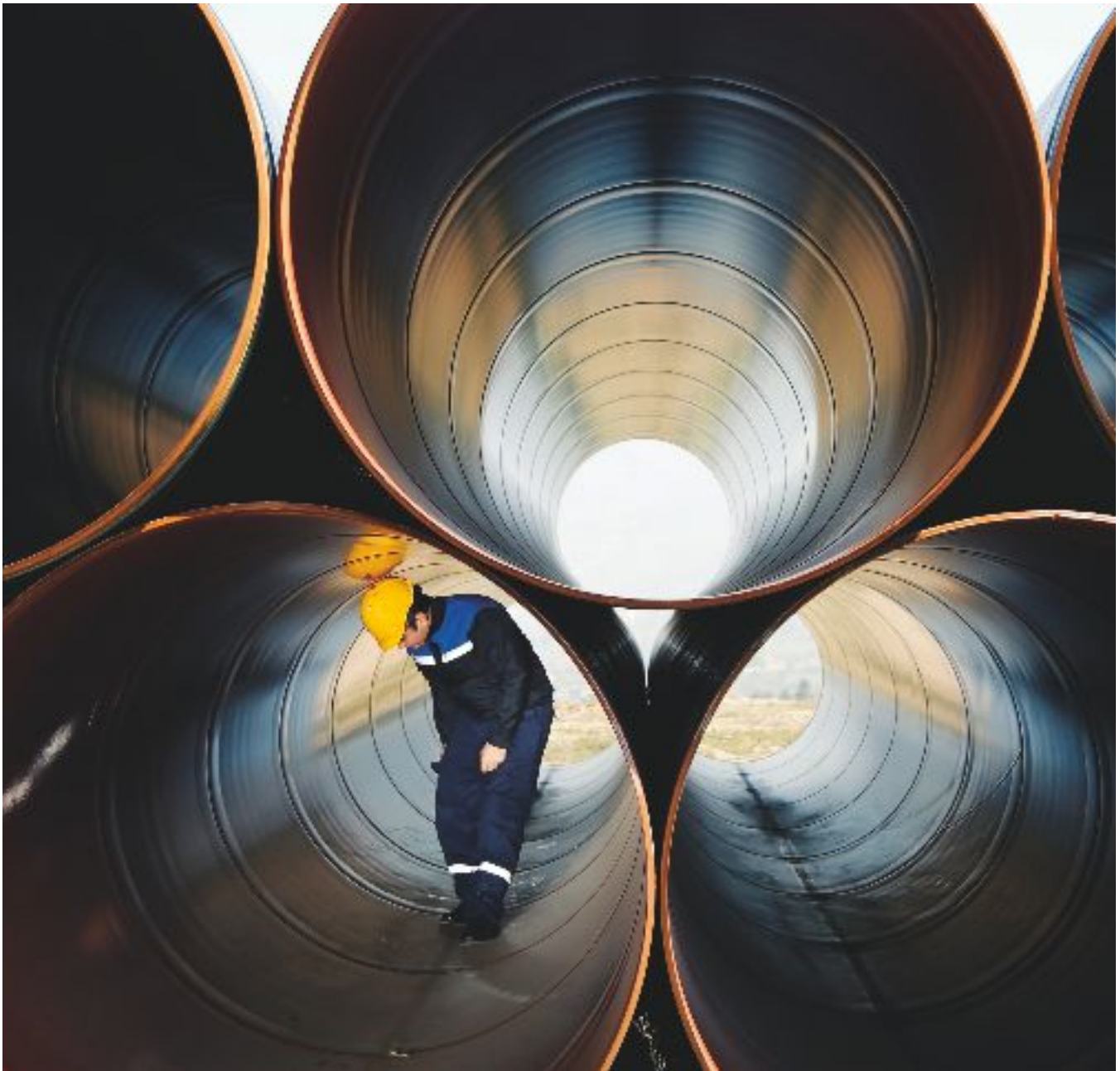
Pre construction pipes close-up view (large diameter)
