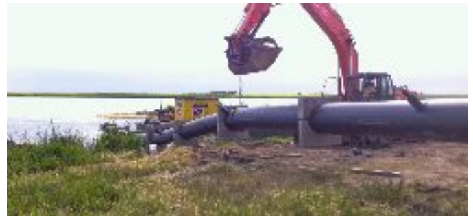
Final Assembly of Reservoir Winter Intake Section
