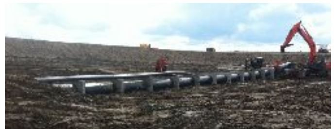
Construction of Intake Lines in Cofferdam
