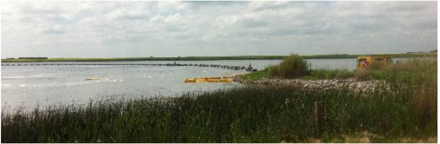
Winter Intake Moving to Installation Position
