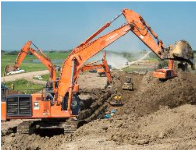
Installation of 750 mm Diameter PVC Piping
