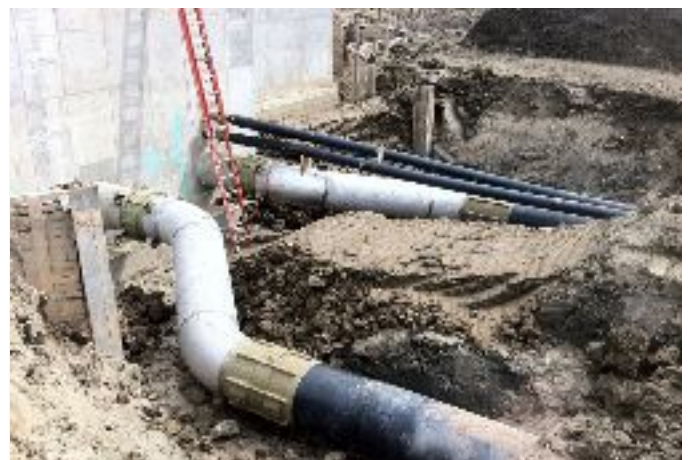
Pump Station Intake Pipes Construction
