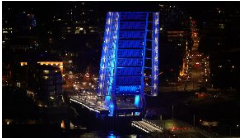
Nighttime - showing the fully illuminated underside of the Orthotropic Steel Deck (OSD)
