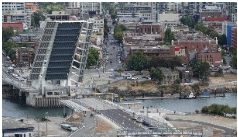
New Bridge in raised position after removal of “Old Blue” showing the west side approach span, western plaza areas, connecting walkways and new pedestrian bridge (foreground).
