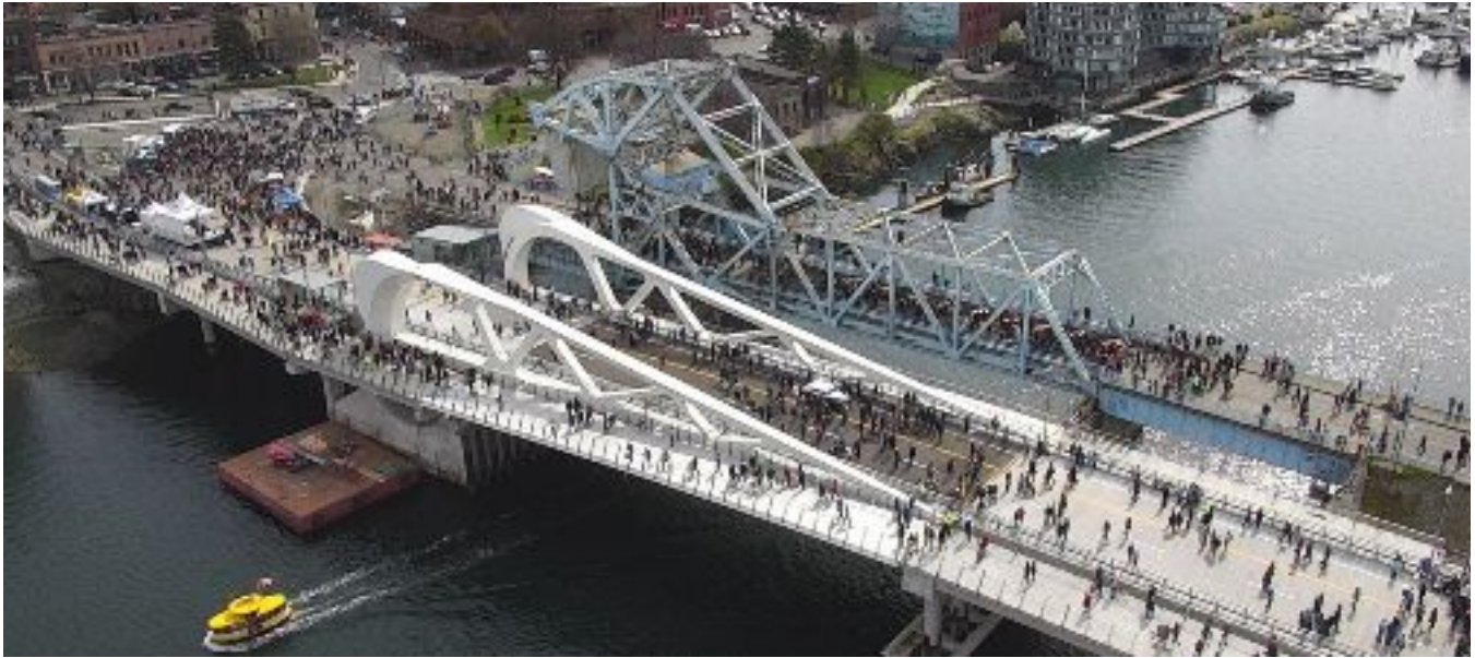
New Johnson Street Bridge on opening day in comparison to original bridge
