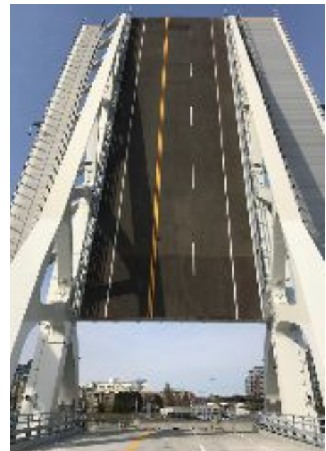
New Johnson Street Bridge in 'open' position
