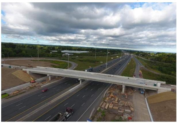
The design life of the new structure is 75 years and in accordance with the Canadian Highway Bridge Design Code (CHBDC). To ensure the long-term durability of the structure we followed the requirements of the MTO Structural Manual and specified premium corrosion protection materials such as stainless steel and Glass Fibre Reinforced Polymer (GFRP) reinforcing bars where required.
