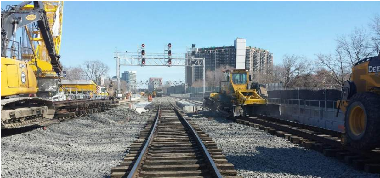
Figure 3: Track panels connected to the west following span replacement.
