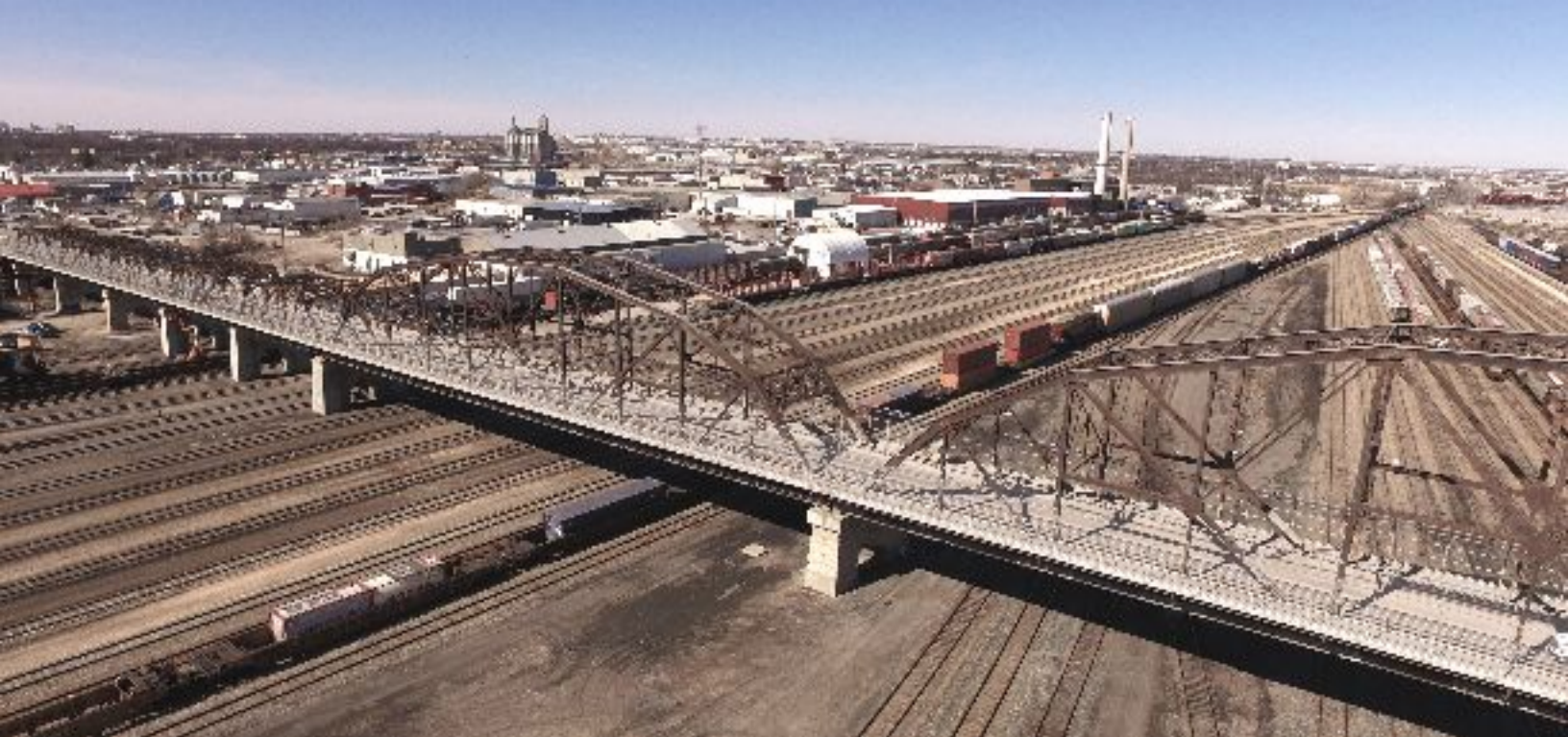
Arlington Bridge Looking Southwest
