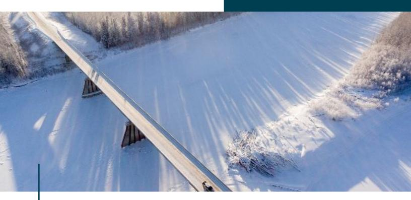
The new bridge is longer than three soccer fields and has five spans that are each 50-76m long, as well as approach land spans about 35m each.
