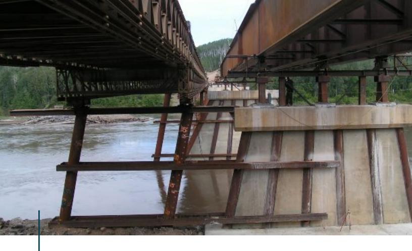
The overhead incremental launch of the steel girders meant no interference with the river below.
