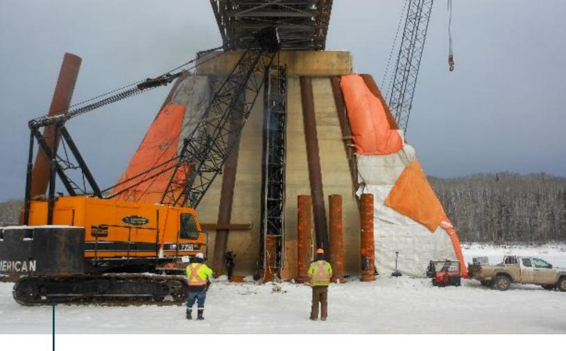
The ice bridge is a sustainable construction methodology. The platform allowed workers to access the substructure for the retrofit, and to store cranes and equipment.
