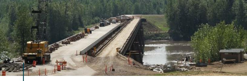
McElhanney devised a traffic staging scheme whereby the existing superstructure was slid 10.5m onto temporary pier extensions to serve as a traffic detour.
