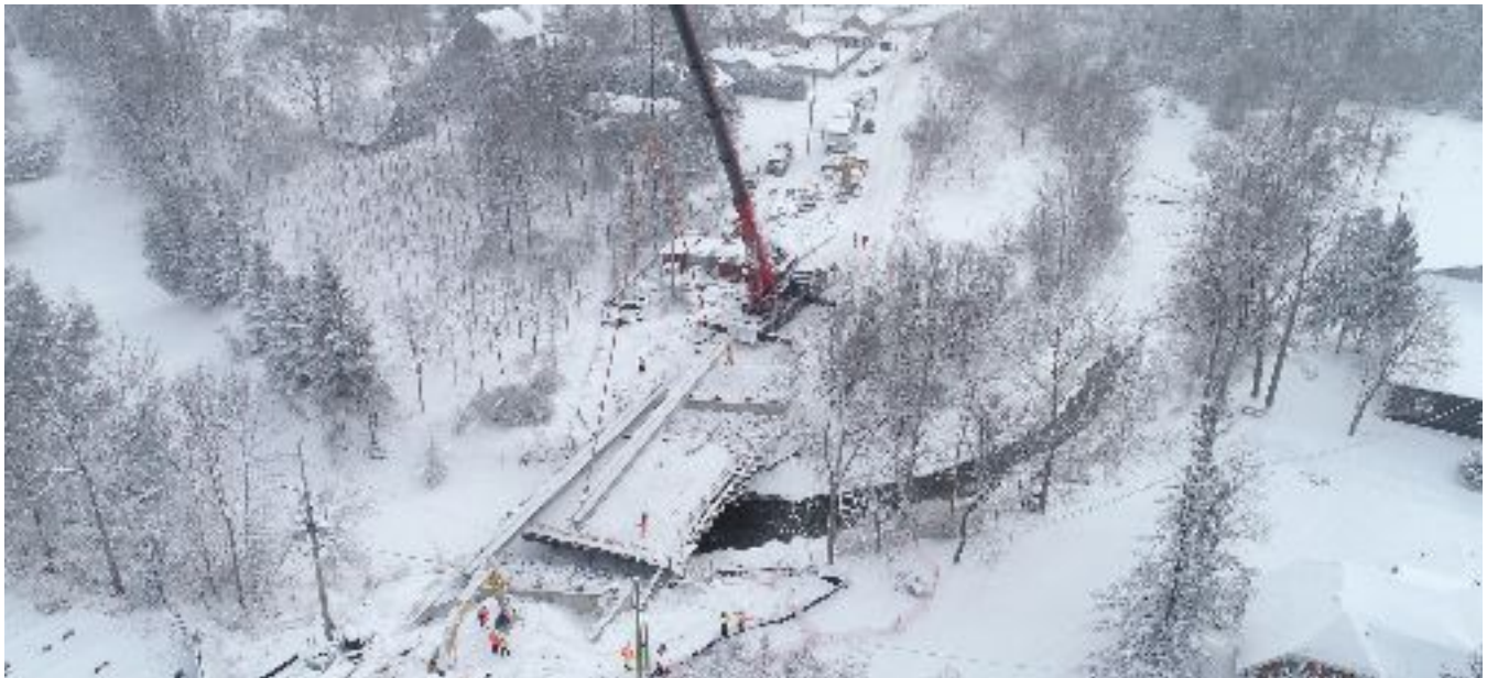
Erection of Girders
