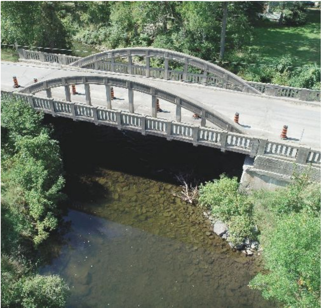
Overhead view from east
