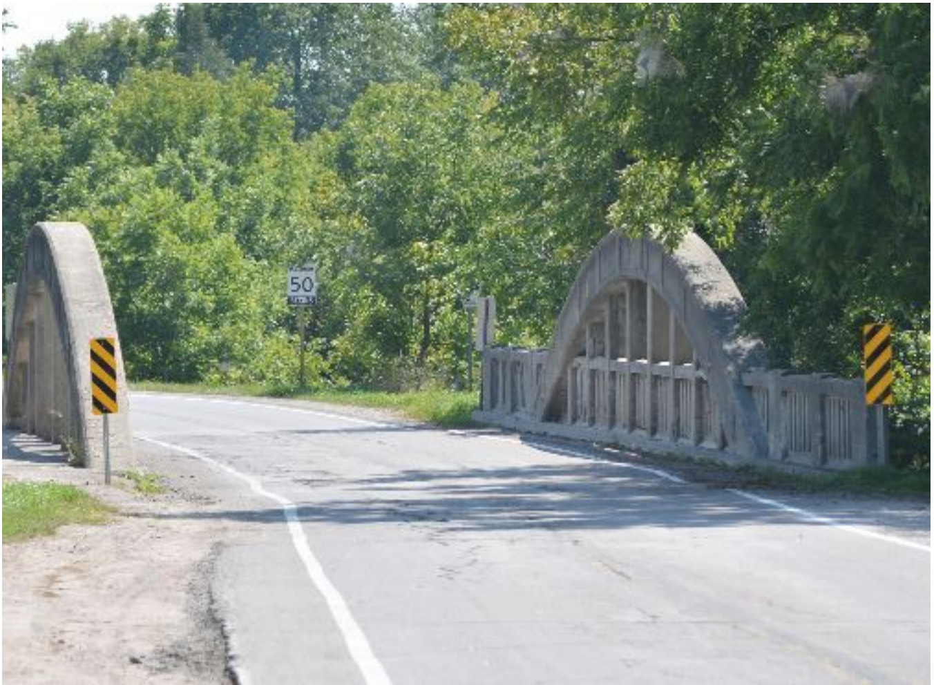
Looking south at bridge
