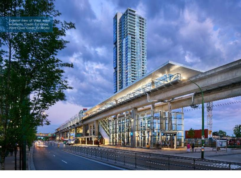
ast + Epp was the structural engineering firm for an ambitious expansion of Metrotown Skytrain Station in Burnaby, British Columbia. The result was a fully modernized station which more than doubled in length from 80 meters to 200 meters, with all work being achieved while the station remained fully operational.
