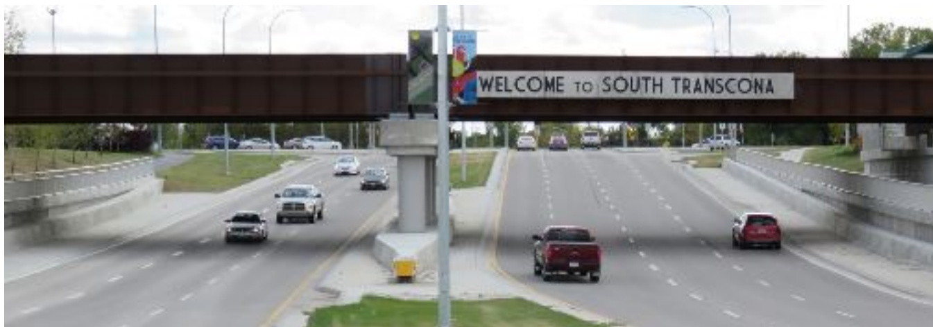
Plessis Road Underpass - Looking South
