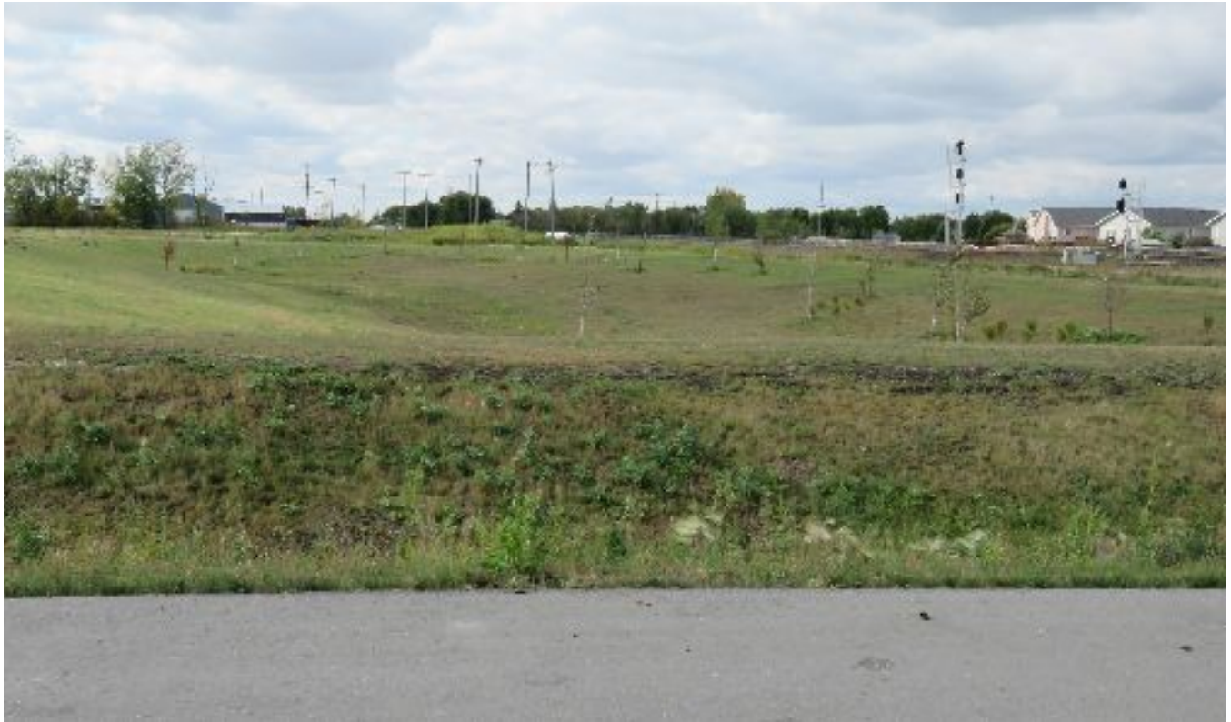
Dry Retention Pond
