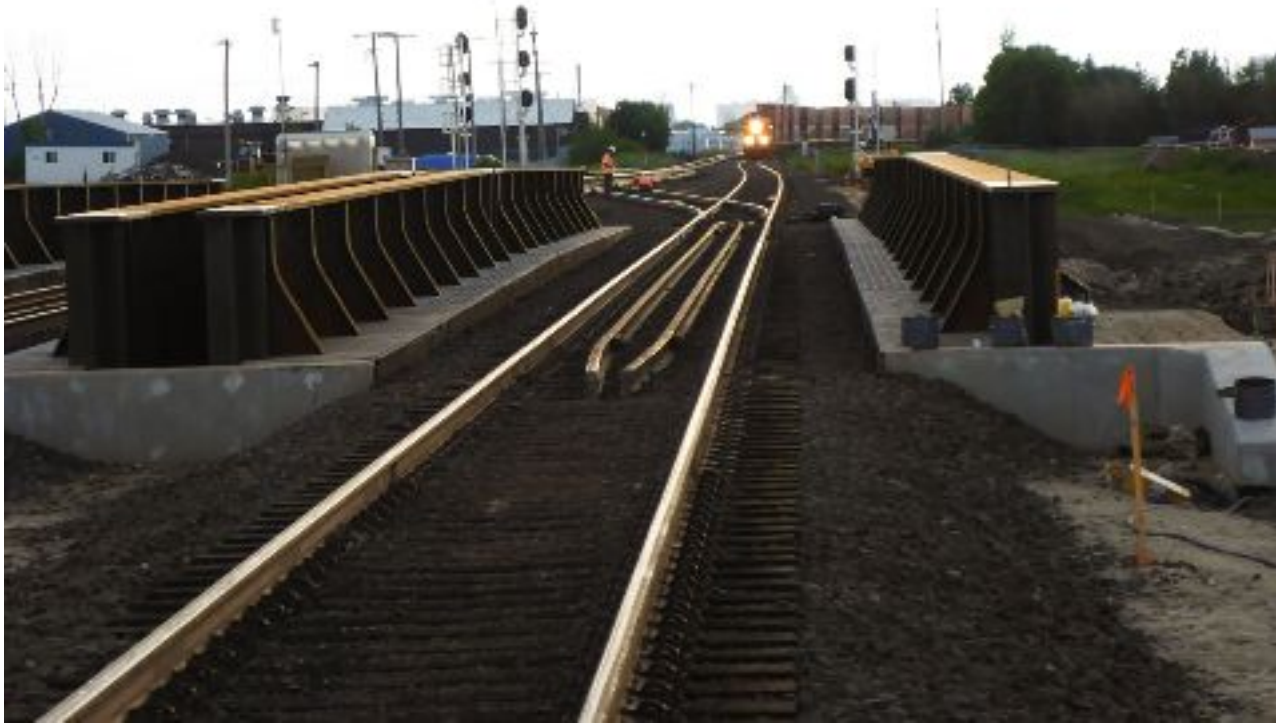
First Train to Approach Bridge after North Track Cutover
