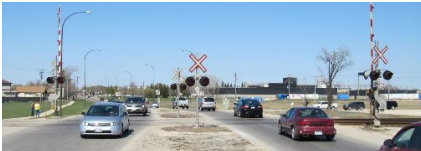
At Grade Road Crossing – CN Redditt Subdivision at Plessis Road
