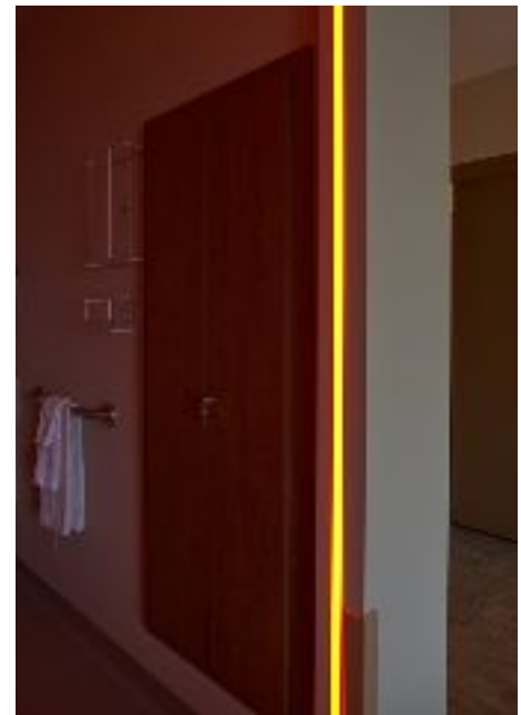
Figure 9. View of Door LED Strip
