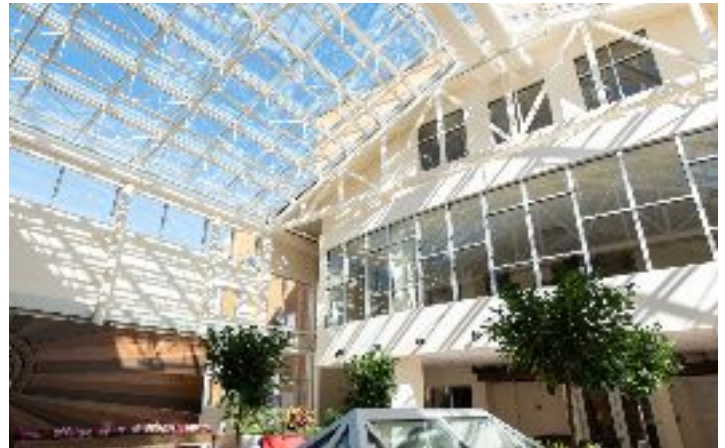
Figure 3. View of Atrium
