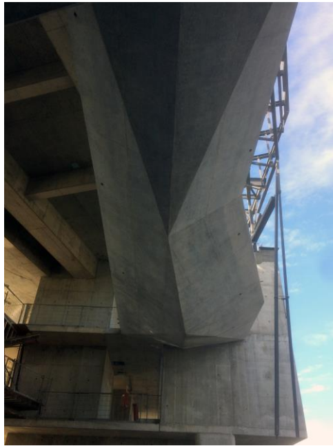
BRIDGE LOUNGE CONSTRUCTION.
