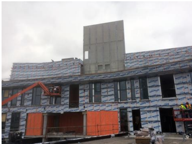
SOLAR WALL CONSTRUCTION AND OPEN SOLAR CHIMNEY. Photo credit: Baird Sampson Neuert Architects Inc.
