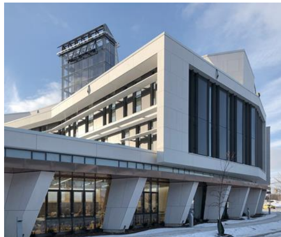
SOLAR WALL CONSTRUCTION AND OPEN SOLAR CHIMNEY. Photo credit: Baird Sampson Neuert Architects Inc.
