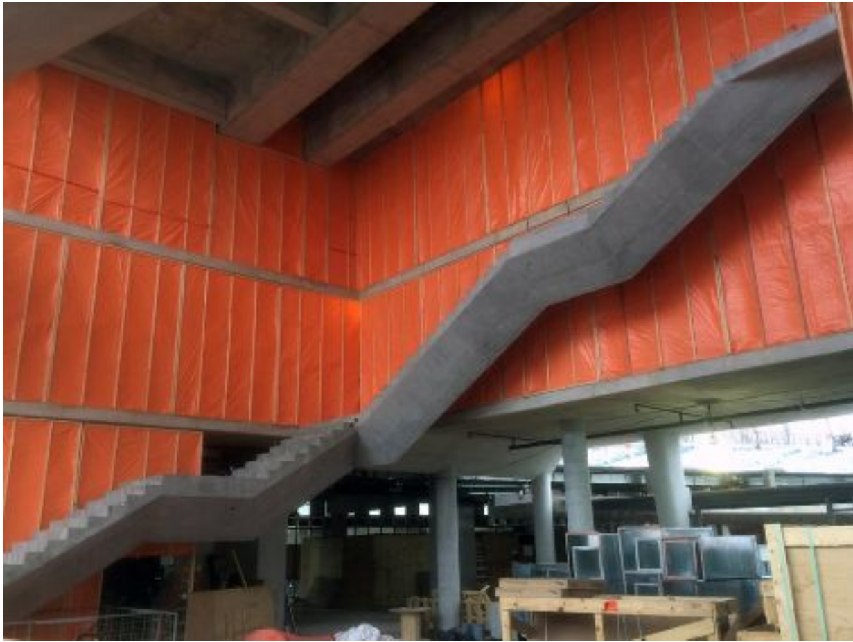
CONSTRUCTION OF FEATURE STAIR.
